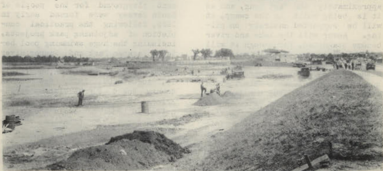
Laying the base for Cooper River Parkway
