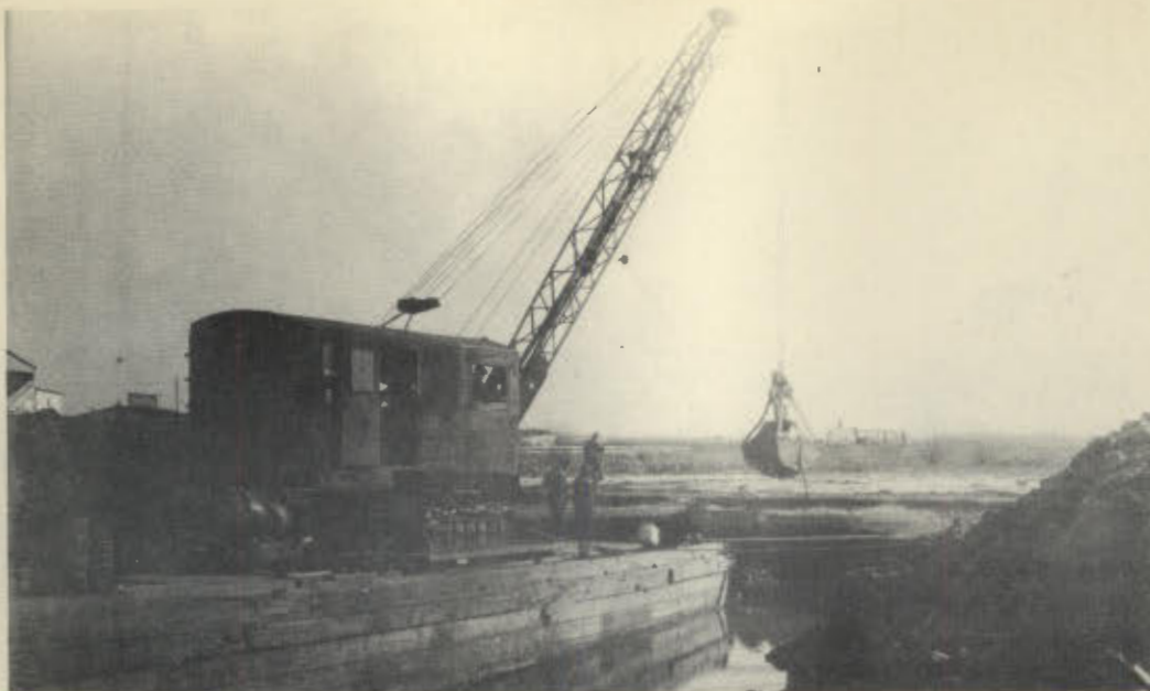
Turning swampland into dry, level ground
