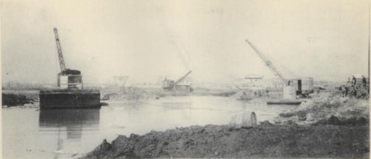
Dredging and excavation at Cooper River, Camden
