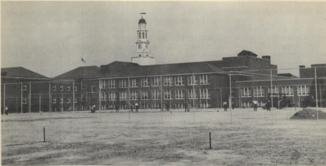
Constructing tennis courts at the Trenton Central High School
