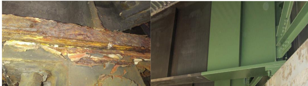
Figure 1. An Over-coated beam: US Route 202 over NJ Route 29 before and after Over-coating
