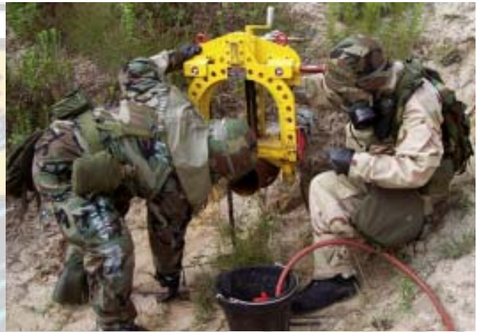
177th Liquid Fuels Airmen repair a fuel line in 80 plus degree heat. Photo by Tech. Sgt. Robert Campbell, 823RED HORSE.
