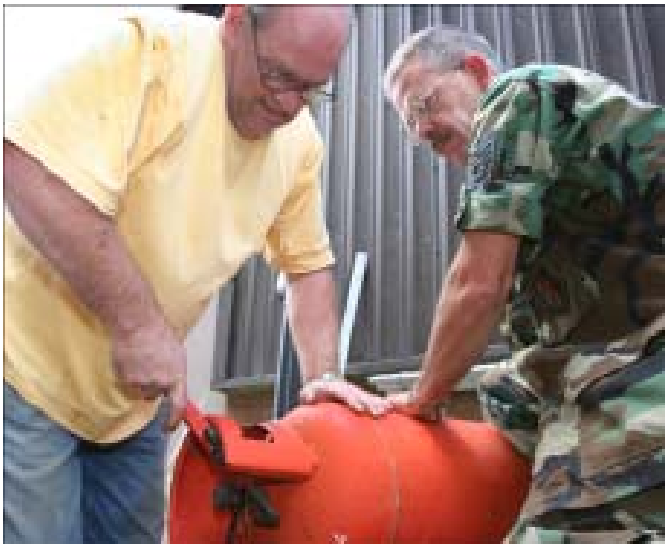
Geoff Harrison (left), RAF Mildenhall Heating, Ventilation and Air Conditioning and Tech. Sgt. Ernie Scott (right) remove a nozzle on gas bottle.
