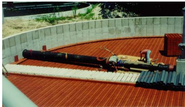
PHOTO COURTESY OF CAMERON ENGINEERING & ASSOCIATES, LLP NEW TRICKLING FILTER UNDER CONSTRUCTION
