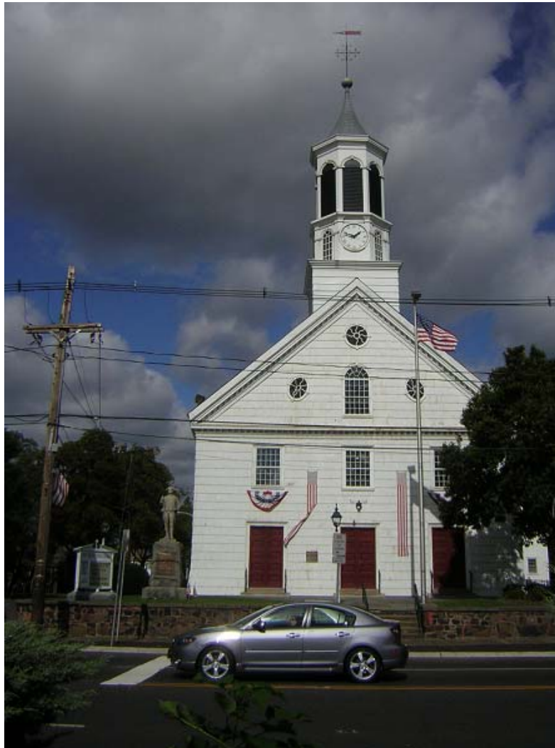
Figure 12: Presbyterian Church in Springfield Source: Photograph by the Author
