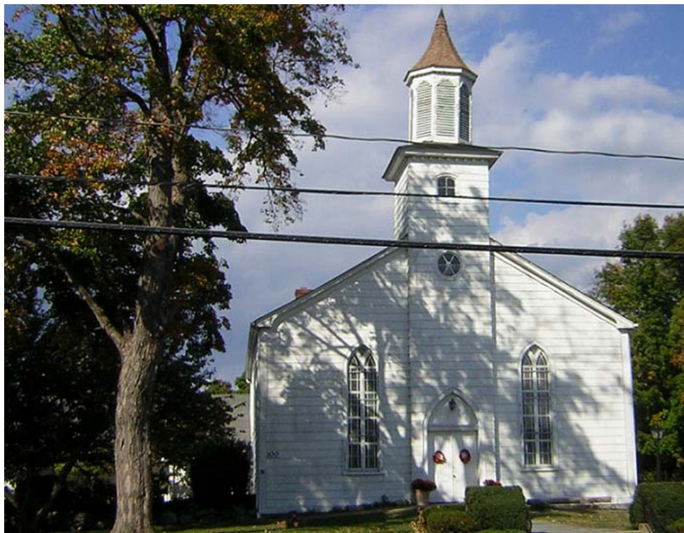
Figure 64: Ramapo Reformed Church Source: Photograph by the Author
