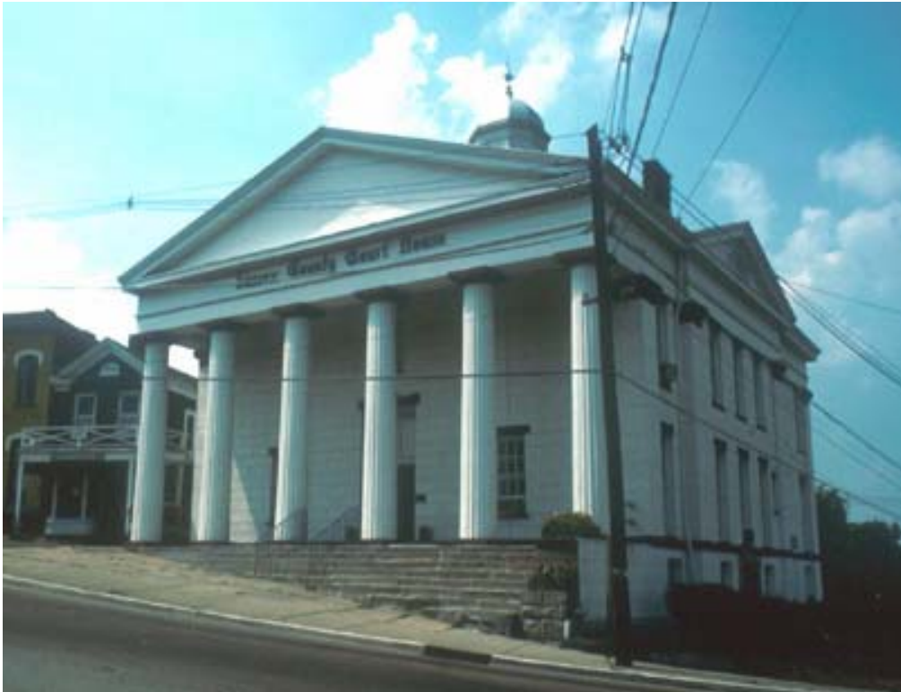
Figure 111: Sussex County Courthouse Source: Photograph by the Author
