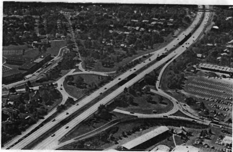
Garden State Parkway Exit, Clark
