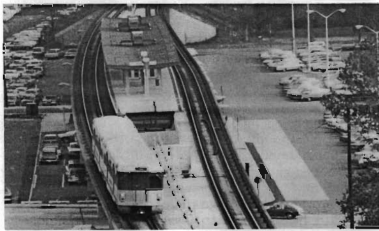
Lindenwold High Speed Line at Westmont Station
