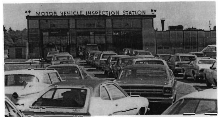
Motor Vehicle Inspection Station, Route 1, Lawrence Township
