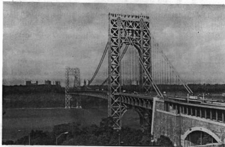
George Washington Bridge, Looking Toward New Jersey Palisades
