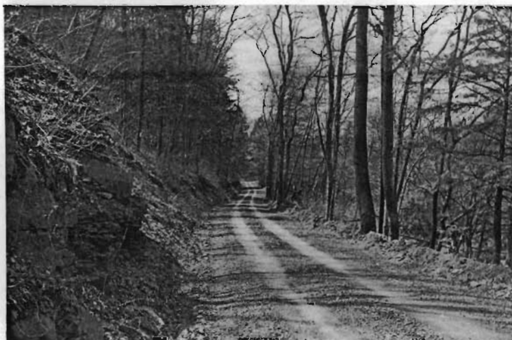
Early Improved Road near Frenchtown
