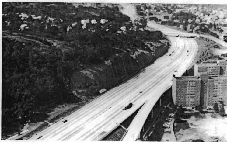
Construction of Interstate Route 80 near Garret Mountain, Paterson
