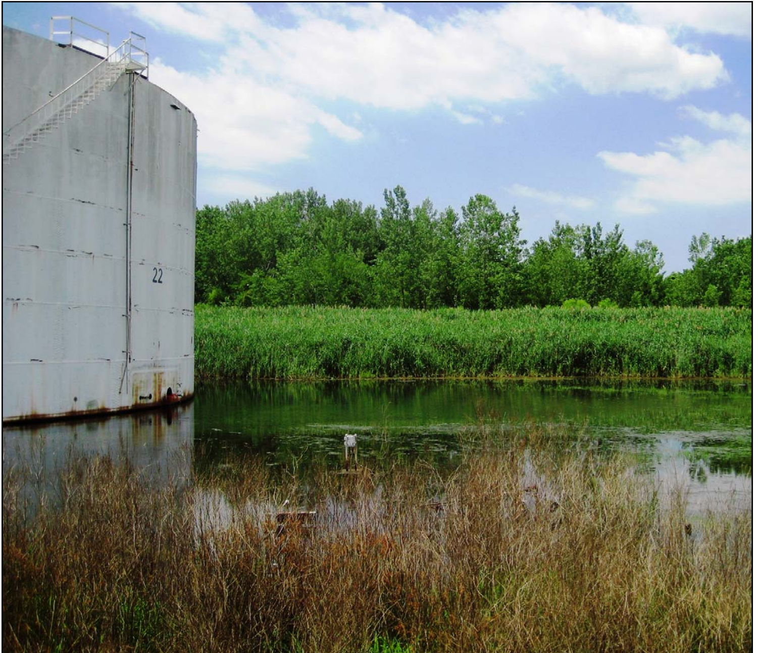
CITGO oil tank sitting in a detention area that may succeed to wetlands habitat
