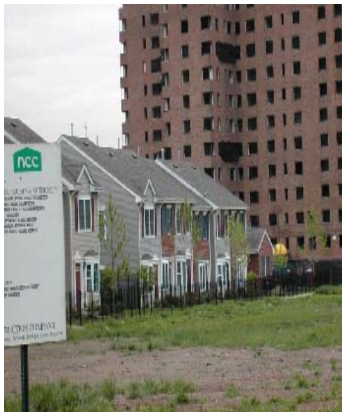
Community Hills Townhouses, 206-unit development in Newark's south ward. In the background is an old public housing development that the City will demolish. --photo by Chester Chinsky, New Jersey Department of Labor
