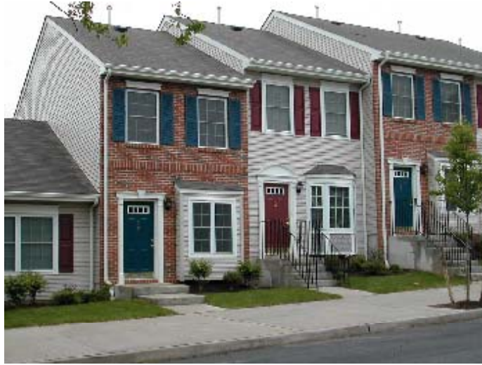
Community Hills Townhouses, Newark south ward --photo by Chester Chinsky, New Jersey Department of Labor
