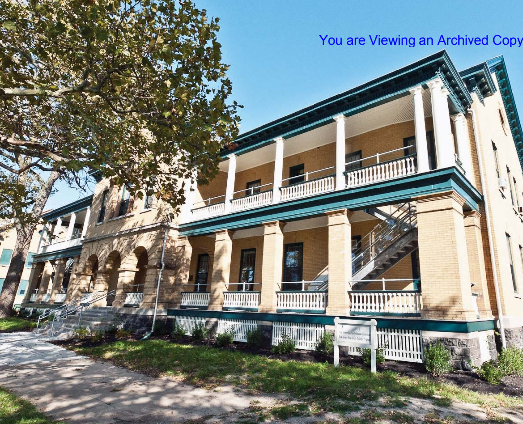
Barracks Building Number 22 at Fort Hancock, Sandy Hook.
