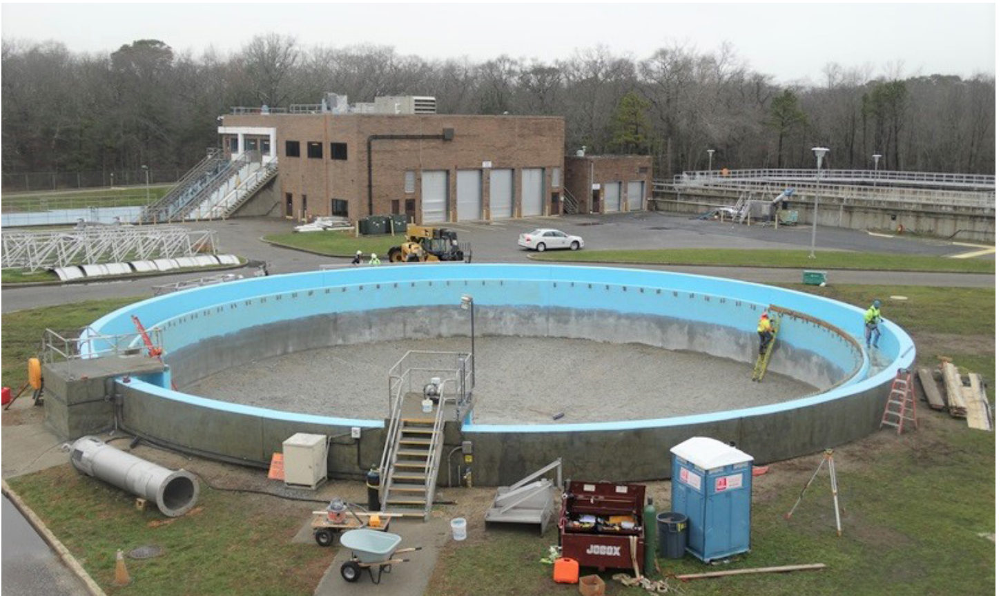
Ocean County Utilities Authority, Clarifier Tank Rehabilitation. SFY2017 Loan: $6,211,590
