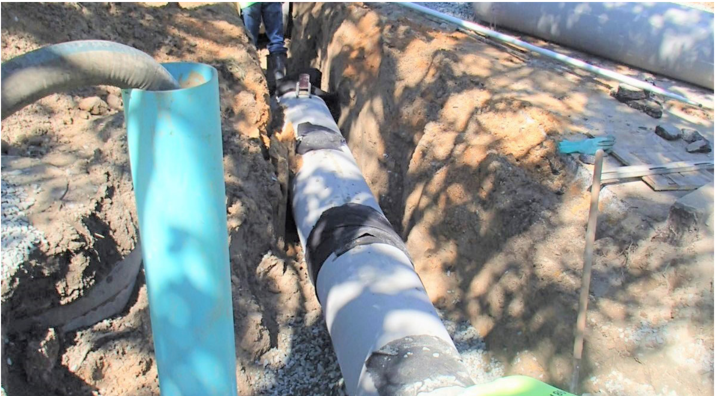
Hammonton Town, Water Main Replacement. SFY2017 Loan: $691,936
