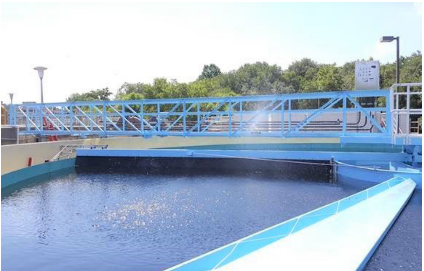
Millville City, Clarifier Tank Upgrade. SF2017 Loan: $9,539,463
