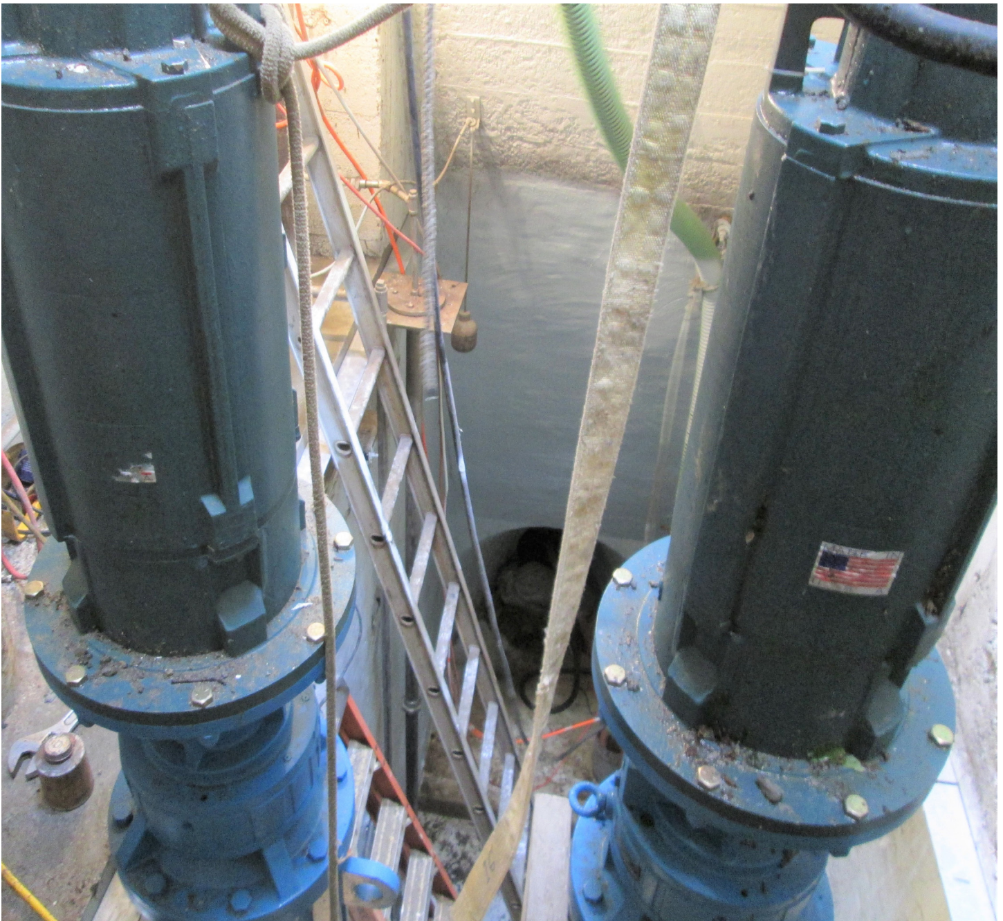
Passaic Valley Sewerage Commission, Yantacaw Pump Station Rehabilitation. SFY2017 Loan: $3,030,000
