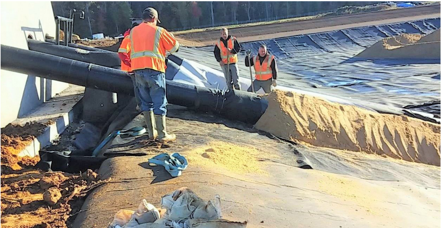
Salem County Improvement Authority, Landfill Cell Expansion. SFY2017 Loan: $5,628,700
