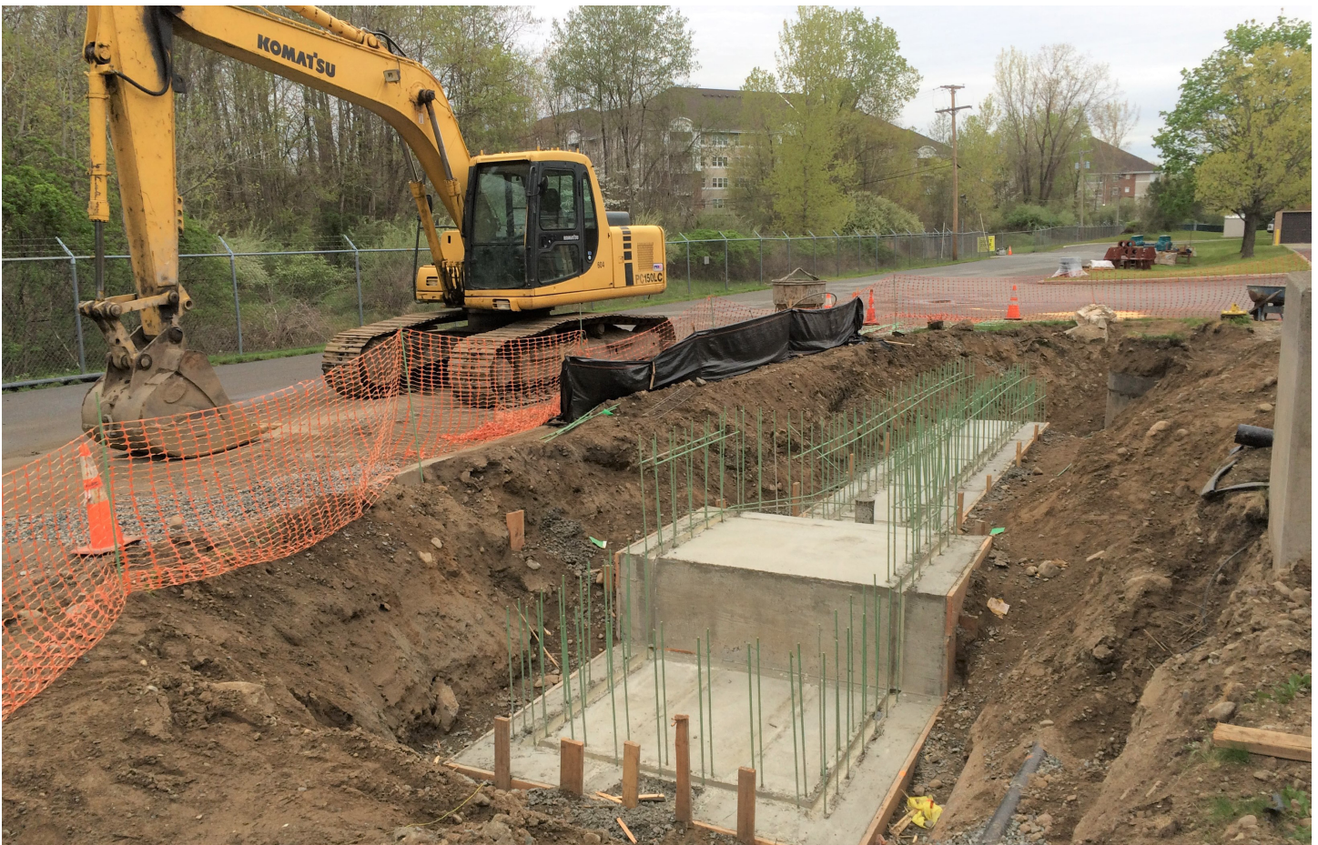
Wannaque Valley Regional Sewerage Authority, Back-up Generator Pad Foundation. SF2017 Loan: $1,360,524
