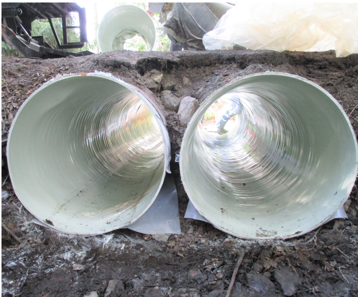
Burlington County, Storm Sewer Relining and Replacement. SFY2017 Loan: $1,710,869
