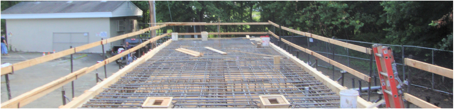
City of Newark, Pequanock Water Treatment Plant Rehabilitation. SFY2017 Loan: $9,347,880.00
