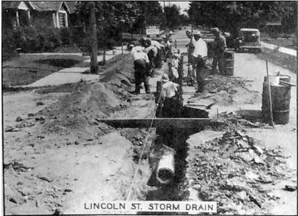
Figure 2. WPA Storm Drain Project in Hackensack, NJ Source: New Jersey WPA, Lincoln St. Storm Drain (The Dawn, September 1936), 6. https://livingnewdeal.org/projects/fairmount-storm-sewers-hackensack-nj/
