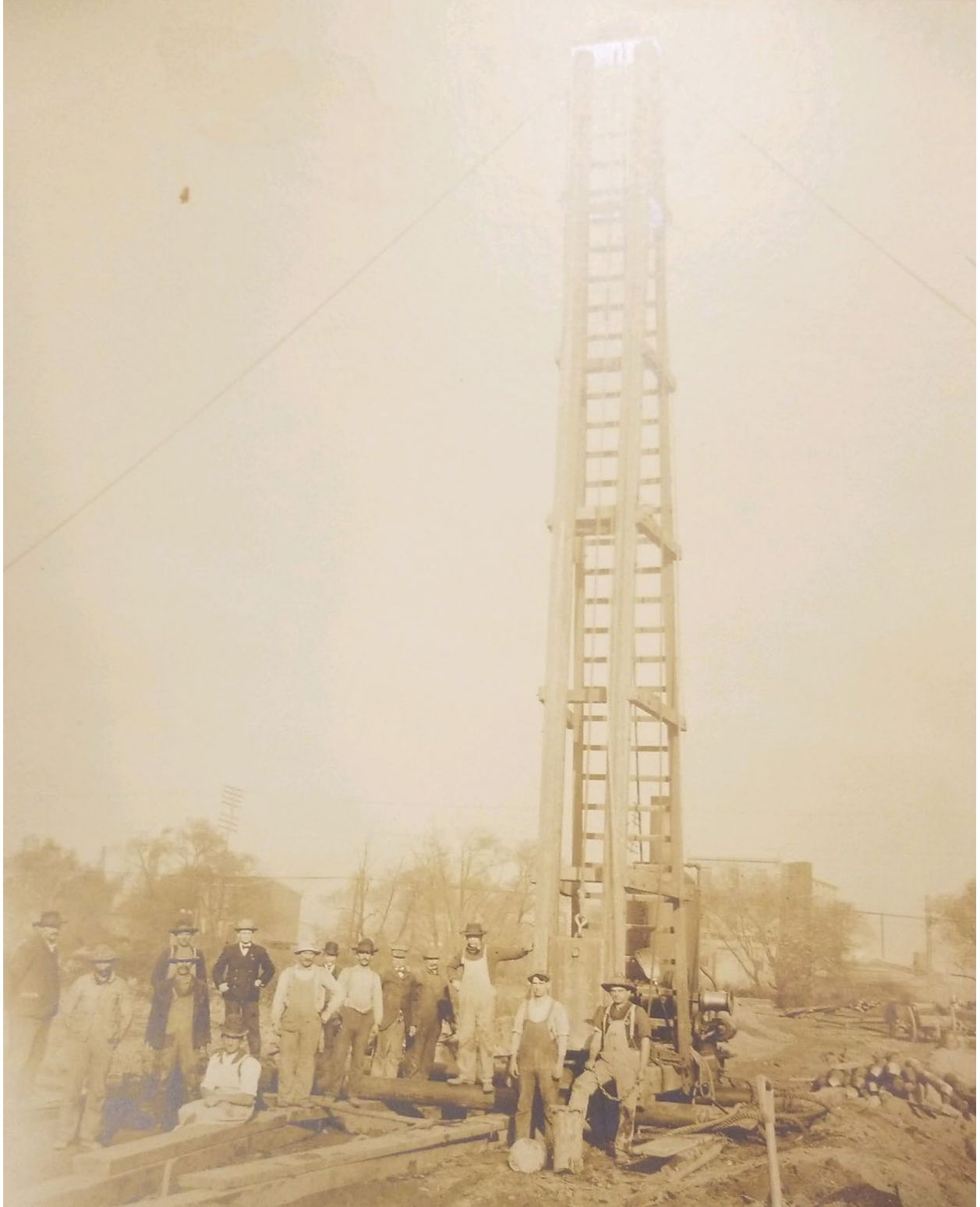
Figure 40. Newton Creek Line Ditch Source: Camden County Historical Society, No. 5015
