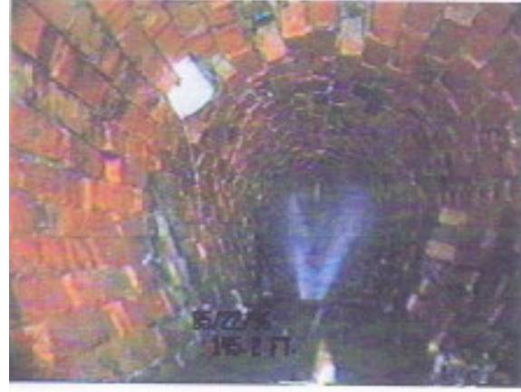
Figure 52. Brick Sewer under Liberty Street, from Haddon Ave to Green Street Source: WRC/D&B Environmental Engineers, Sewer Reconstruction Project, Various Locations City Wide, City of Camden, New Jersey, Project No. S340641-01, (WRC/D&B Environmental Engineers, 2001).
