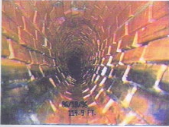
Figure 51. Brick Sewer under 9th Street, from Pearl to Vine Source: WRC/D&B Environmental Engineers, Sewer Reconstruction Project, Various Locations City Wide, City of Camden, New Jersey, Project No. S340641-01, (WRC/D&B Environmental Engineers, 2001).
