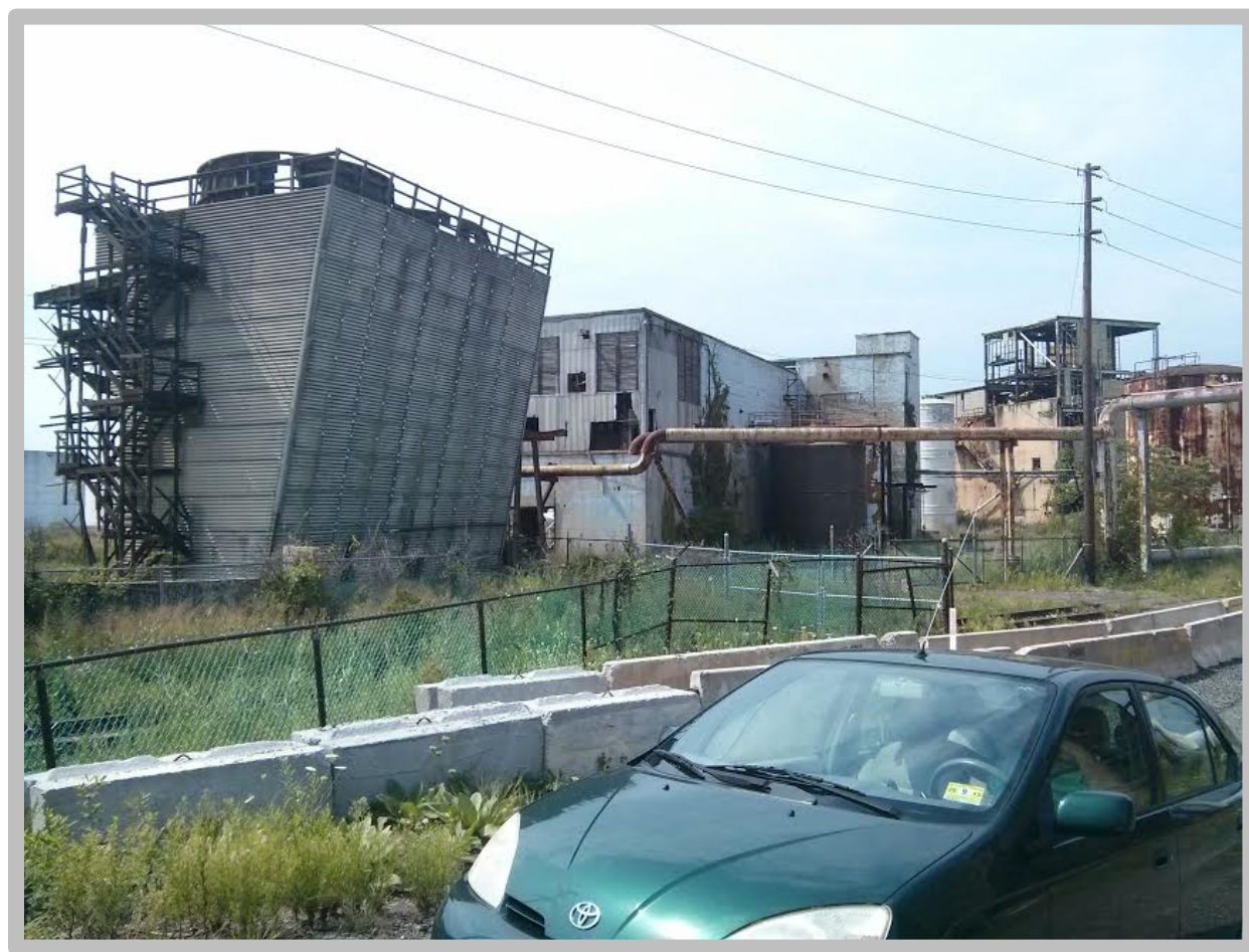
Figure 4. View of the LCP Chemicals, Inc. (LCP) Superfund site
