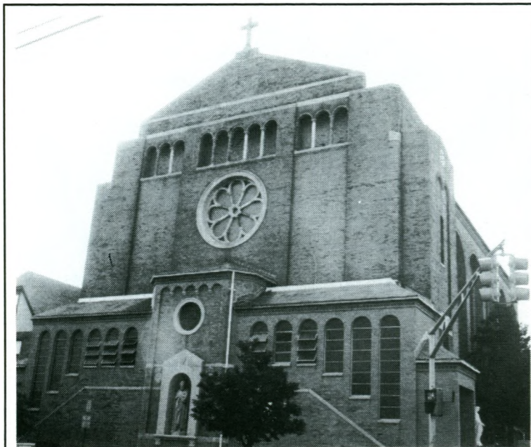
St. John's R.C. Church - Corner Anderson Avenue & Walker Street- 1994.
