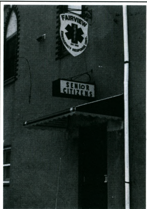
Emergency Response Unit and Senior Citizen Center.
