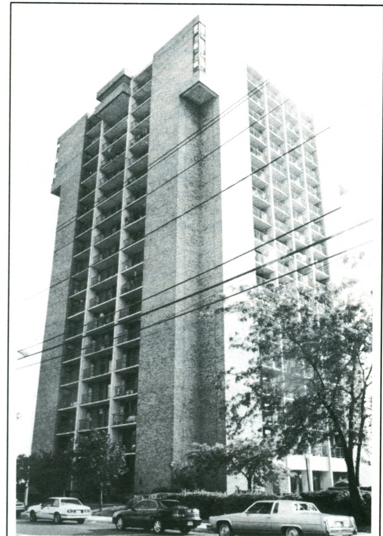
Senior Citizen Building, 370 Fairview Avenue.
