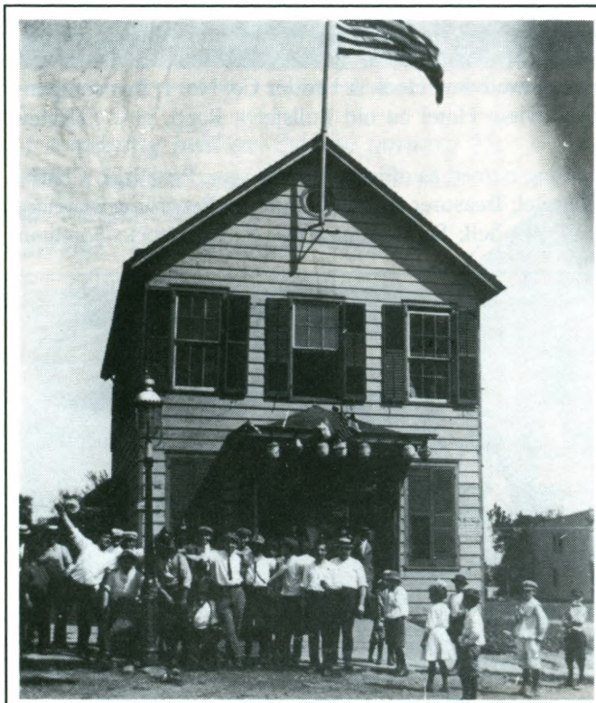
Old Grandview Fire House - Grant Street corner Garfield Street - July 4, 1910 celebration.
