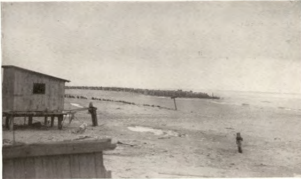
Jetty No. 1. Note pool cutting at end exposing the core. February 4, 1930. Same view as above. Stockade nearly buried.
