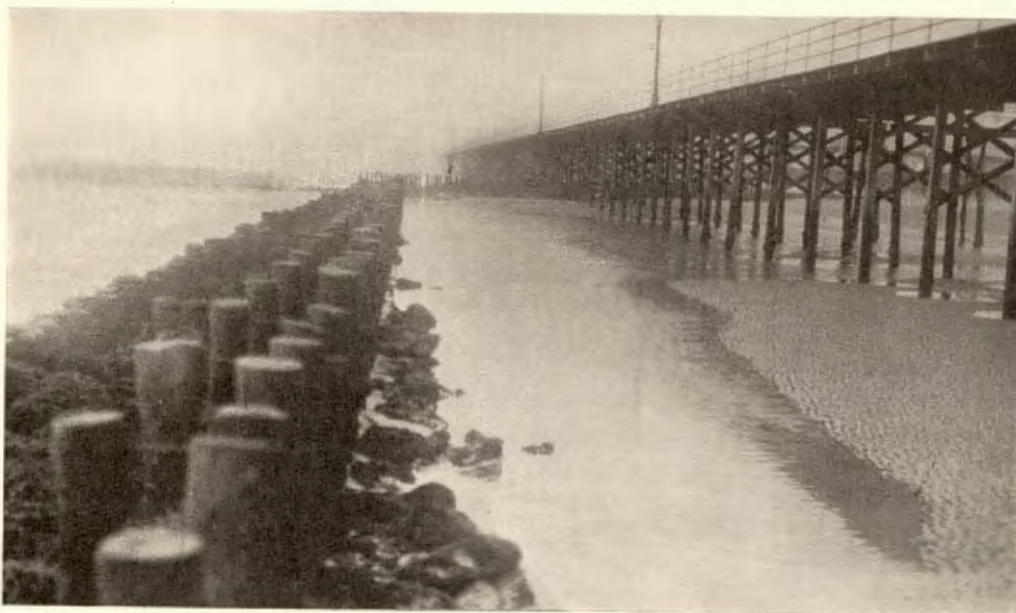
Ventnor Crib Wave-Breaker, July 14, 1928. Depression in right background caused by break in sheeting.
