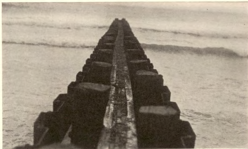
Cape May City, groin of original contract showing steel sheet piling encasement due to attack by teredo.
