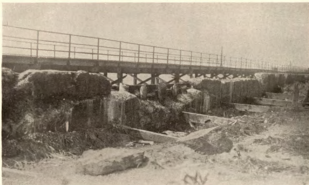
Margate Seawall, July, 1928. Original construction. Concrete deteriorating.
