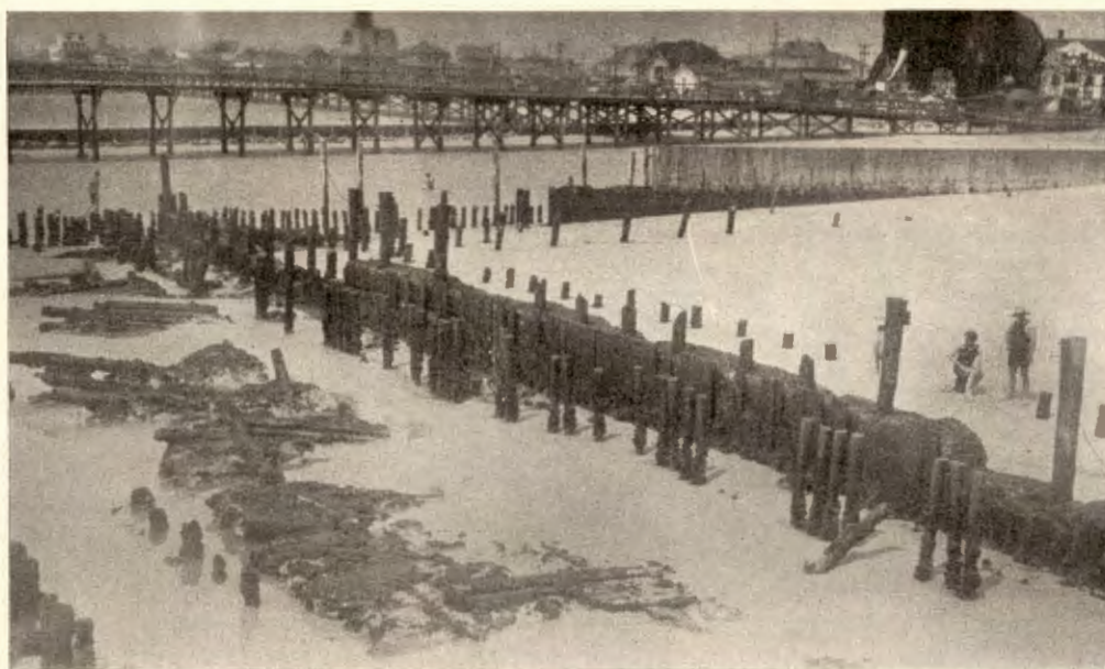
Margate Seawall, July 15, 1928. Note shearing at middle wale.
