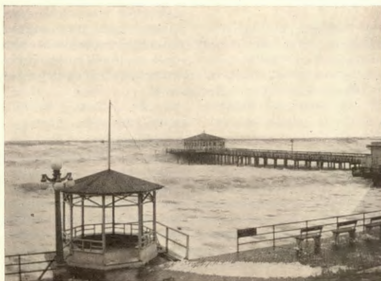
Comber striking floor of pier. February, 1927.
