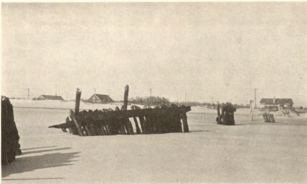
Brigantine City, hook jetties largely destroyed by floating out. February 11, 1930.
