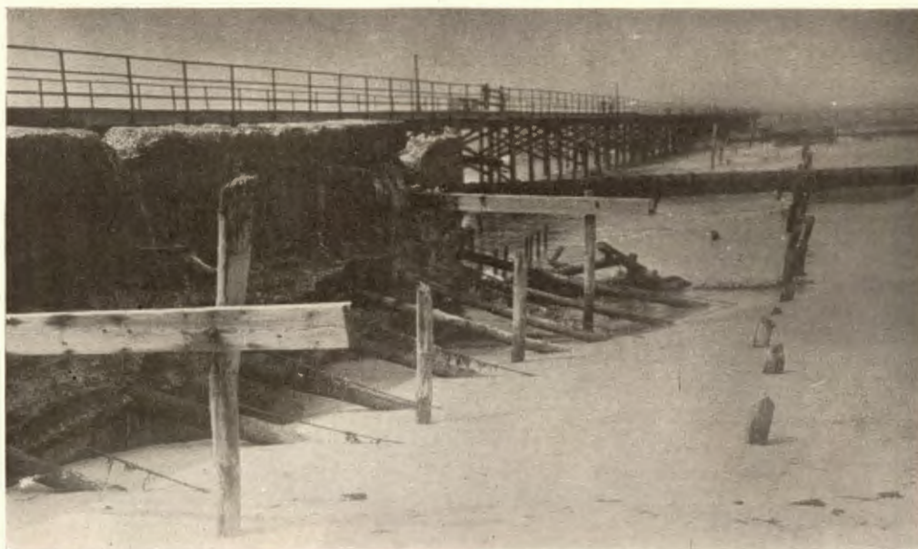
Margate Seawall, remains.
