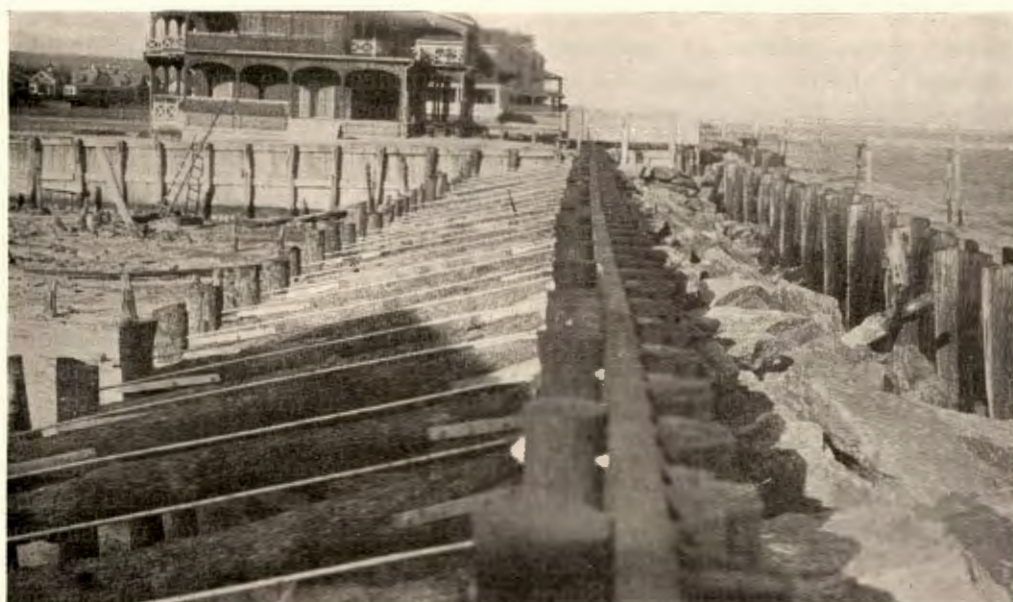
Steel Sheet Pile Seawall, Sea Bright.
