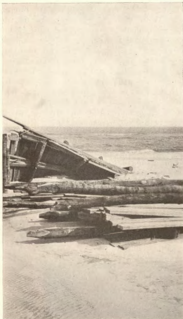
Groin, partly destroyed in place, partly floated out.
