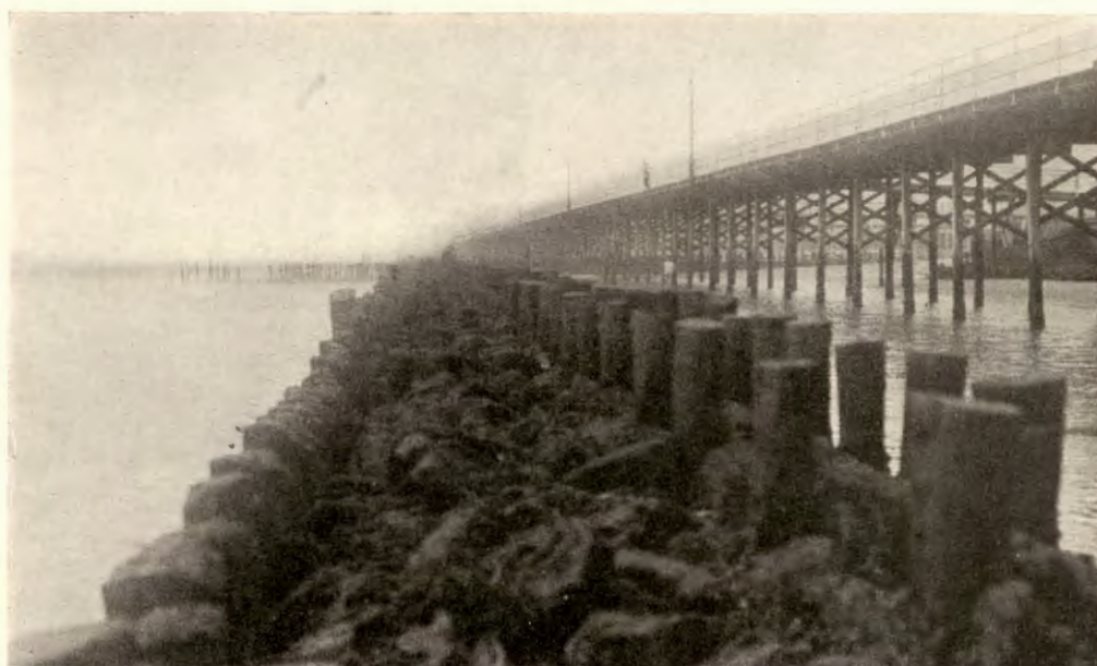
Ventnor Crib Wave Breaker, July 14, 1928. Rock and timber covered by heavy growth of mussels.
