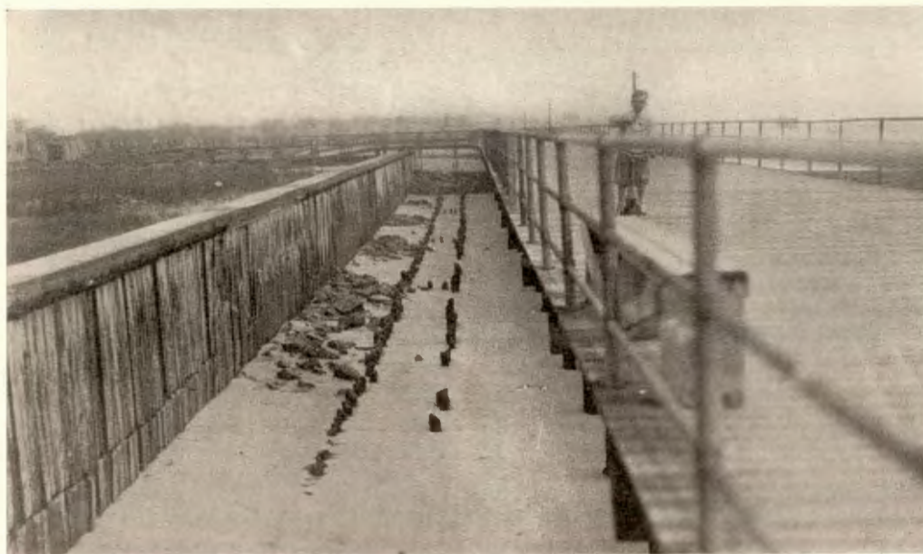
Margate Seawall, July, 1928. Coping replaced with reinforced concrete.
