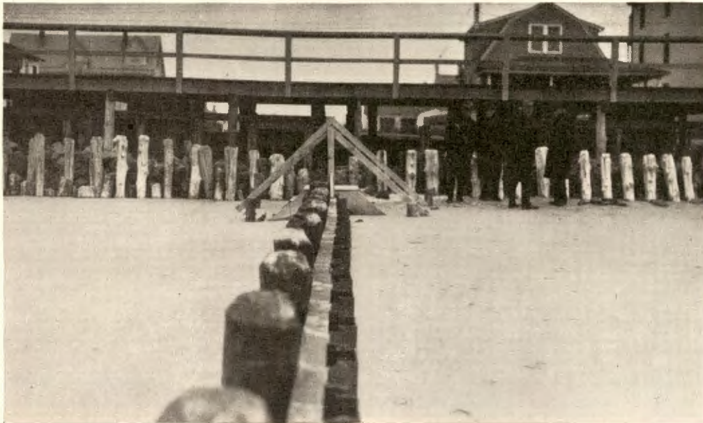
Cape May groin south of Casino showing pronounced accretion. February 27, 1930.
