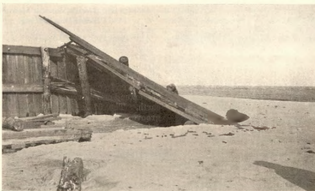
Failure of outer end of groin. Storm of February, 1927.
