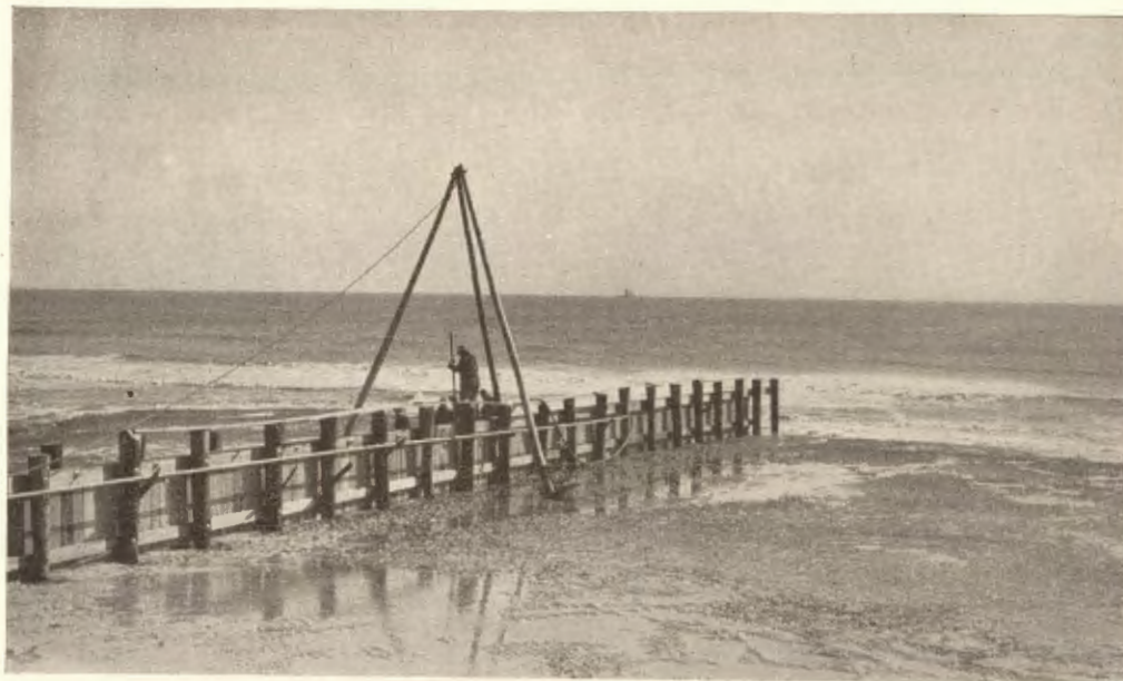
Doubling up piling. Cape May pilot boat is in the distance, February 27, 1926.
