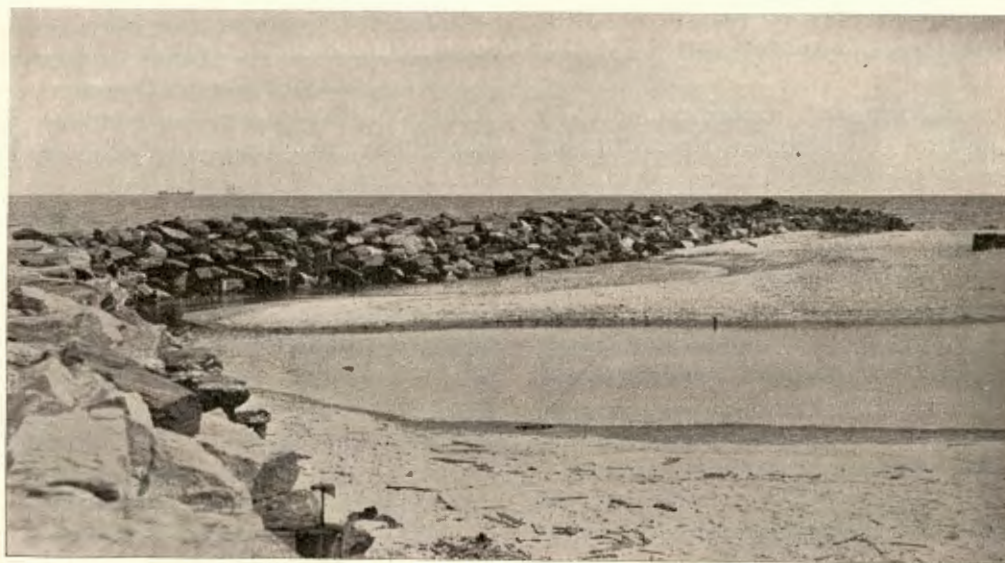
Monmouth Beach jetty showing effect of leaks, September 17, 1927.
