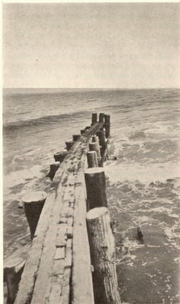
Distortion of outer end of groin.
