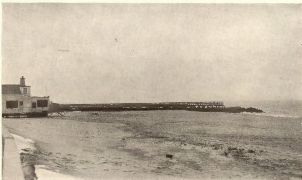
Looking north to Jetty A from inshore projection of Jetty B now almost entirely buried. February 4, 1930.
