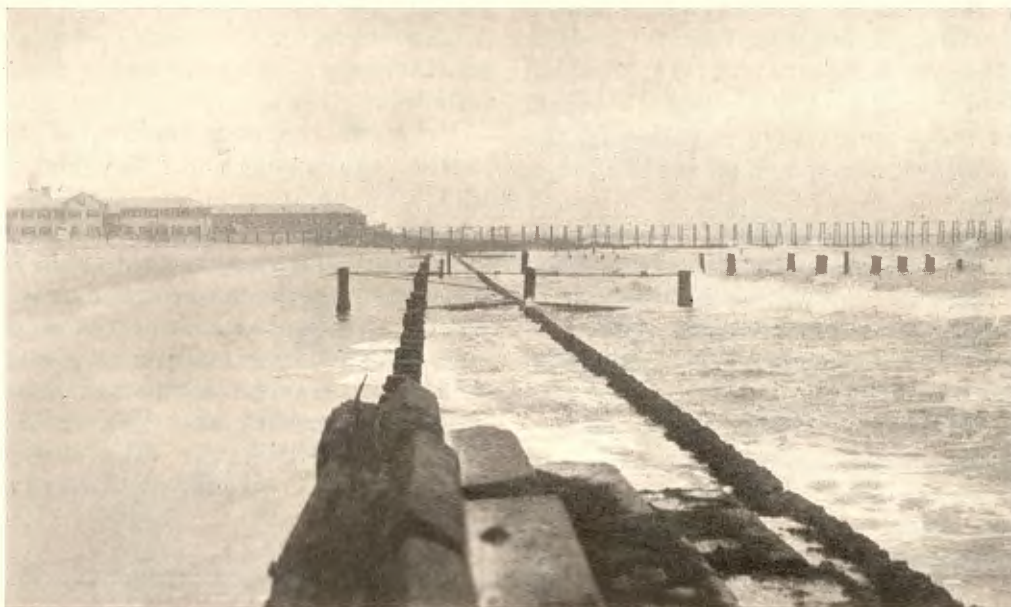
Seawall, Longport, after erosion.
