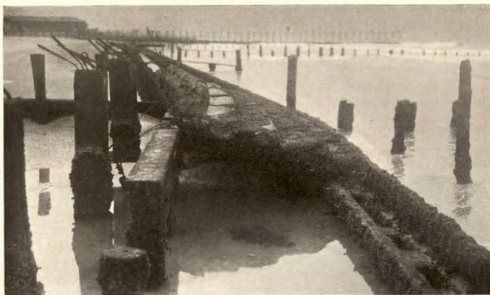
At break, Longport Seawall.
