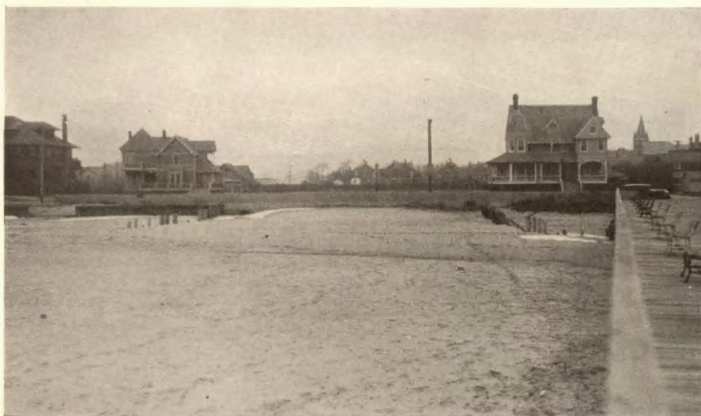
Same view, February 4, 1930. Piling stockade shown prominently in photograph of May 4, 1926, is almost entirely covered.
