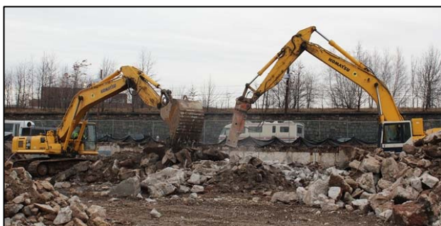
Phase 1 Work at ES #3 site
