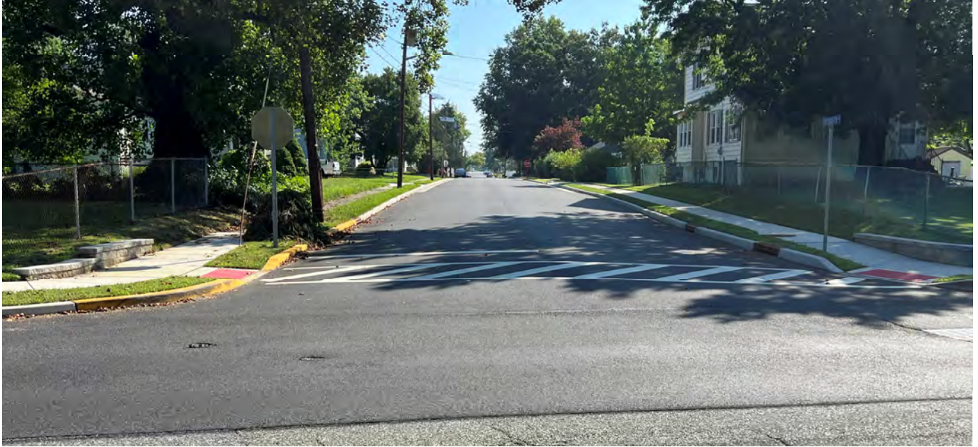
Somerdale Borough Evergreen Avenue Reconstruction. SFY2023 Transportation Bank Long-Term Loan: $8,157,548
