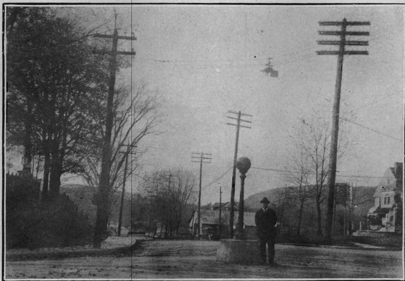
Traffic post with permanent base 4 feet wide placed at intersection of roads. This post may cause accidents or loss of life, for which local officials will be responsible, as it is an illegal obstruction to traffic.
