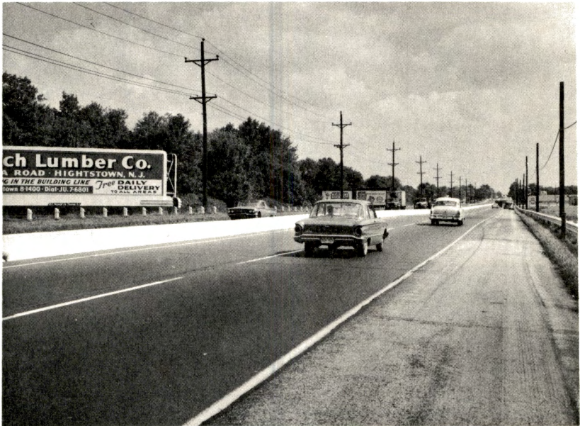
This photo shows completed highway after road has been black-topped and reflectors placed atop the barrier at 100 and 200 foot intervals depending on curvature and topography.
