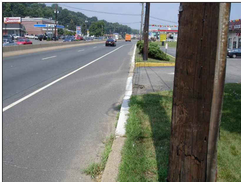
Figure 26. US 22 MP 43.8 Westbound: Pole 62263NPB
