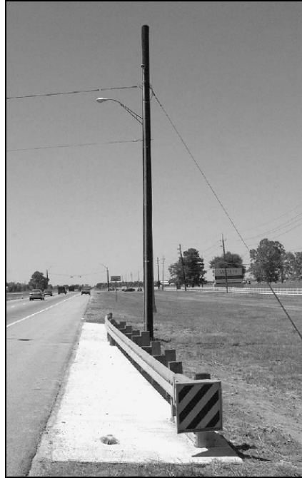
Figure 8. W-Beam Barrier and Extruder Terminal Shielding a Utility Pole [20]
