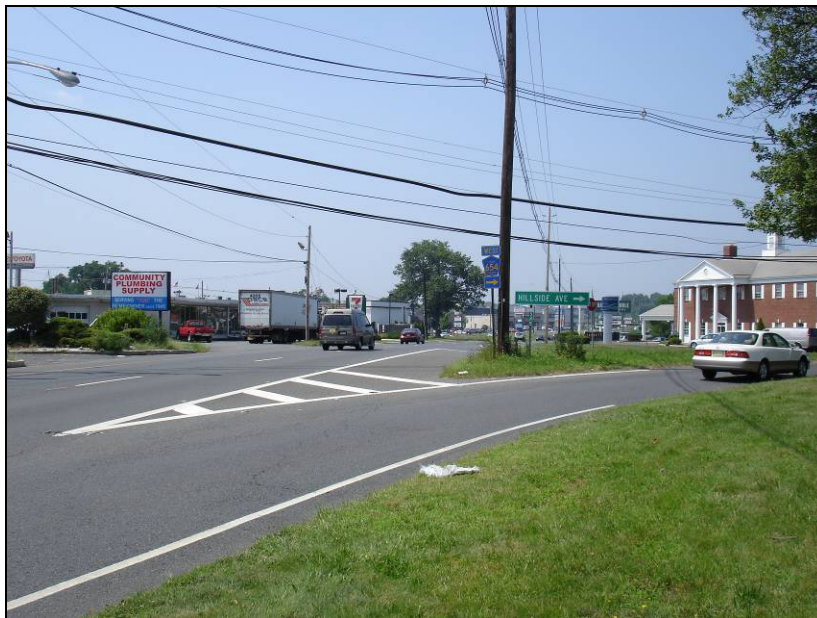
Figure 35. US 22 MP 52.6 Westbound: Pole PS537
