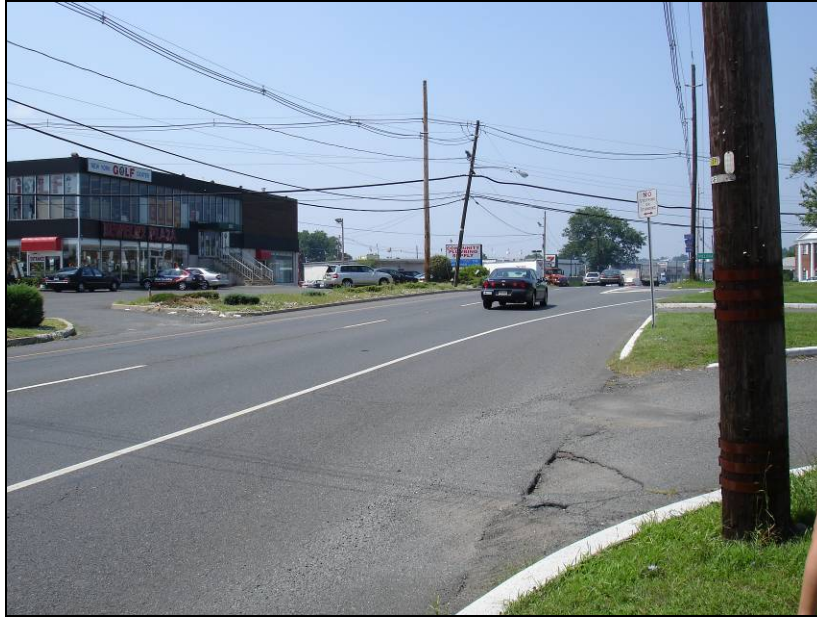
Figure 34. US 22 MP 52.6 Westbound: Pole BT60015SF
