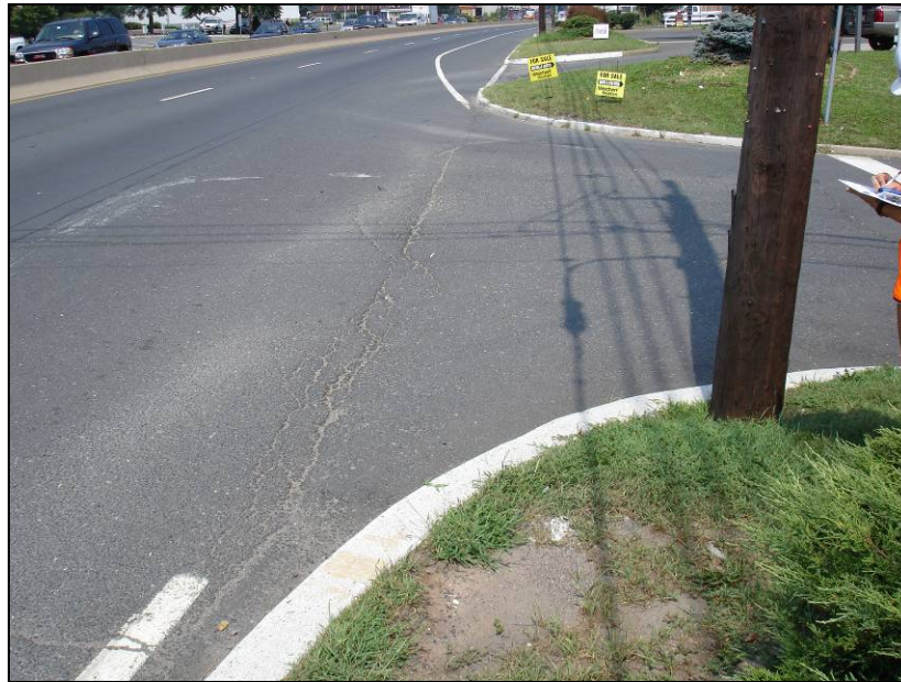
Figure 25. US 22 MP 43.9 Westbound: Pole 61128NPB
