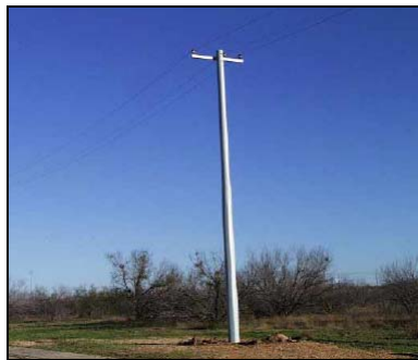
Figure 7. Shakespeare Energy Absorbing Utility Pole
