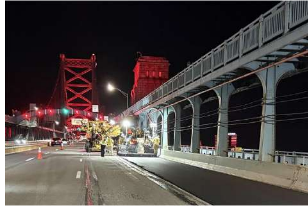
Iconic backdrop, essential work — paving crews resurface the Ben Franklin Bridge overnight.
