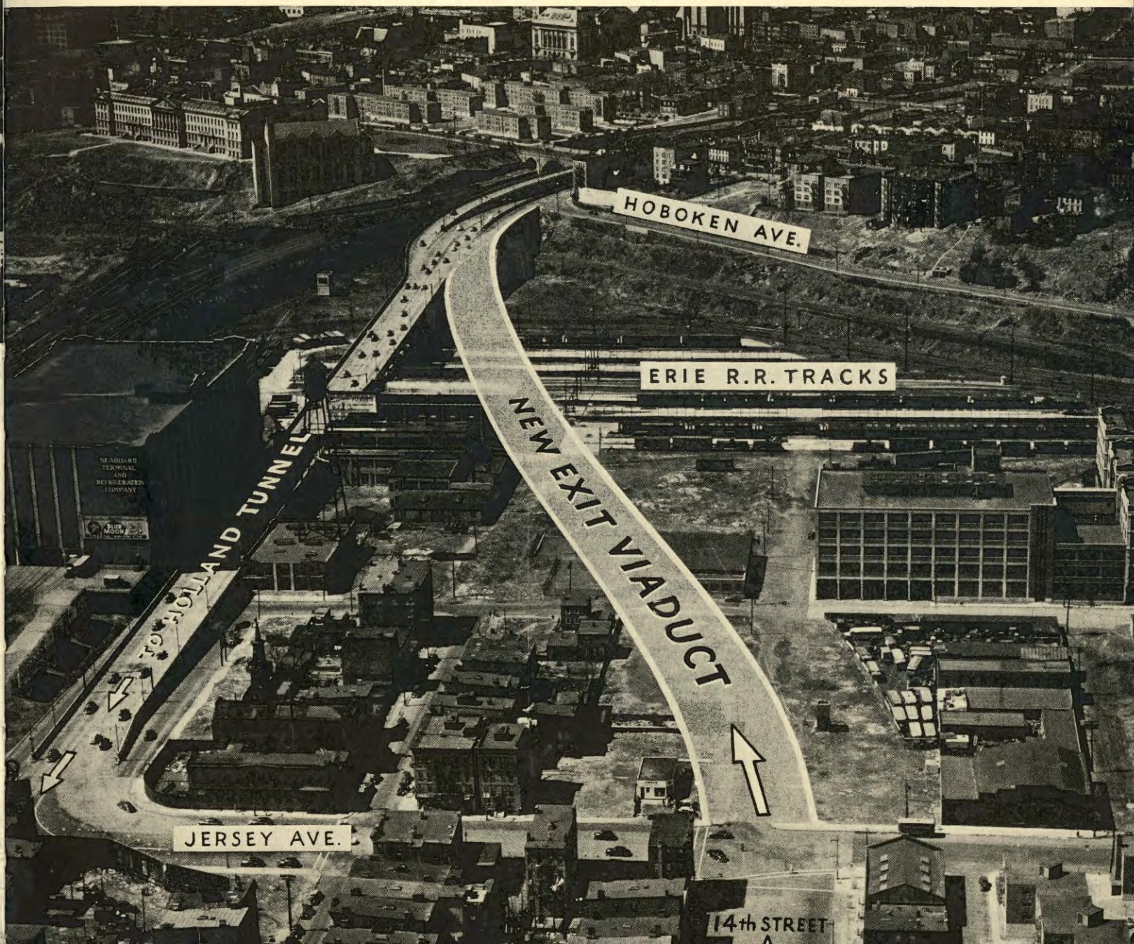
ELIMINATING A BOTTLENECK at the Jersey City exit from the Holland Tunnel. This 2,000-foot-long new Holland Tunnel Exit Viaduct over Erie Railroad tracks to the Pulaski Skyway connection (at top) will eliminate congestion on existing viaduct at left. Heavy Jersey-bound traffic from the Holland Tunnel exit along Fourteenth Street must now make a sharp left turn on Jersey Avenue, then a sharp right to a viaduct carrying two-way traffic. The new Port Authority Exit Viaduct, begun in late 1948, will allow separate streams of one-way traffic with no turns, greatly lessening week-end traffic jams.
