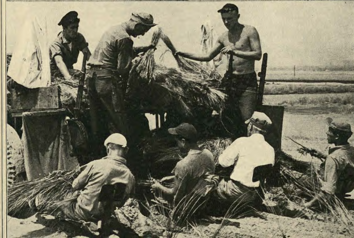
PLANTING beach grass at New York International to stabilize the sand fill and to prevent eroding sandstorms. Effect of the grass after two seasons of spreading growth is to raise the wind level more than six inches above surface of the sand. This tractor-drawn modified tobacco planting machine can plant nearly six acres a day. About 4,000 acres of the airport have now been planted with beach grass ( Ammophila arenaria ), forming an efficient ground cover to control a former serious threat to the airport's usefulness.
