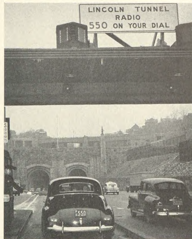
Radio sign at Jersey Plaza of Lincoln Tunnel.
