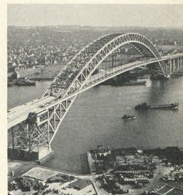
BAYONNE BRIDGE. Port Richmond, Staten Island, to Bayonne, New Jersey.
