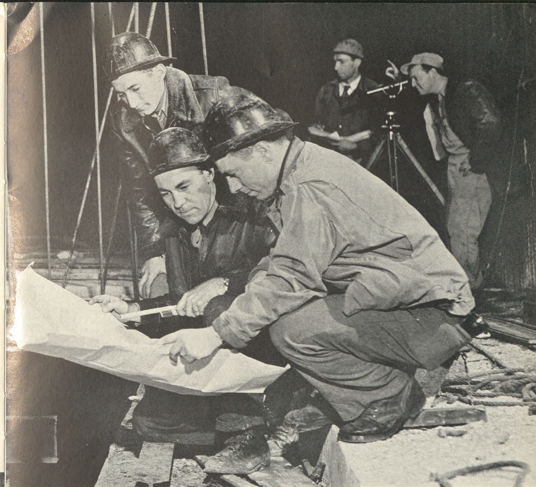
Port Authority engineers check progress of roadway construction at 179th Street Tunnel. Assistant Resident Engineer Tony DeBiase (right foreground) goes over drawings with Inspector Al Weeks (center) and Surveyor Ike Dornfeld, while Surveyors Joe Kelly and Chuck Fagan observe alignment of roadway slab.
