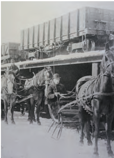
LVRR's coal depot at South Plainfield, New Jersey, circa 1900 (Source: Gary Karasik and Anna M. Aschkenes, Middlesex County: Crossroads of History, 1999).
