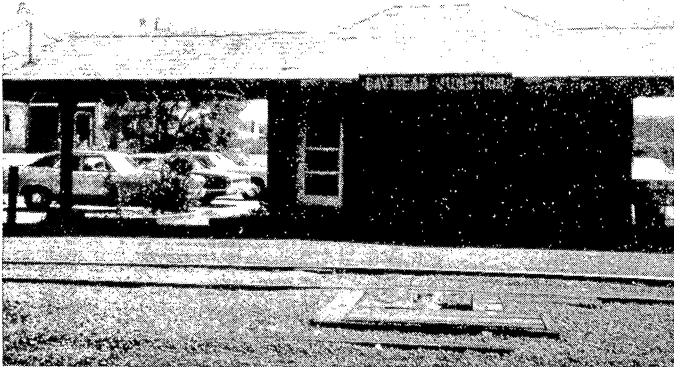
BAY HEAD STATION BUILDING
