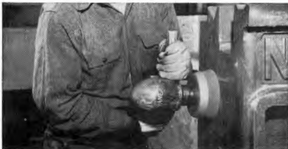
The revolving cup guard is used on either the straight or flaring type cup wheels for off-hand grinding.
