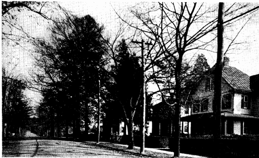
Fig. 11. High Tension Electric Cable Carried Through Street Trees with No Serious Injury Done.
