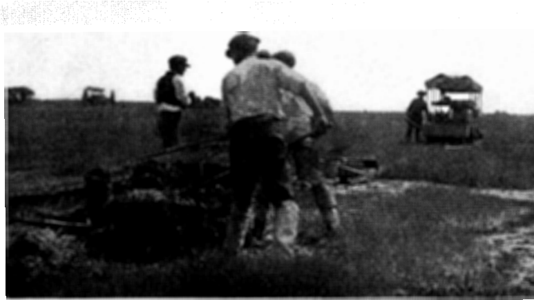
Fig. 15. Cutting a Mosquito Ditch by Machinery.
