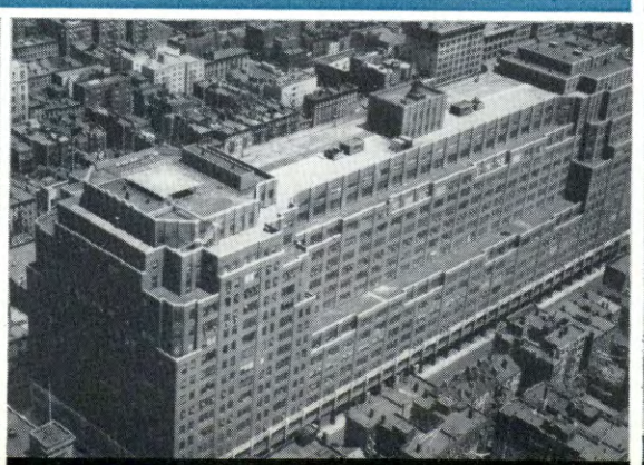
Port Authority Building
