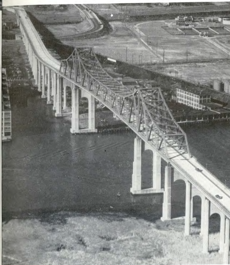
Improvements to Port Authority vehicular crossing approaches in progress at the year's end included the $4,225,000 construction of a connection between the George Washington Bridge and the new Palisades Interstate Parkway, above. Demolition at the New York end of the Bridge preparatory to improving the approach system there is shown, left. Traffic congestion on the Bridge's New York approaches was relieved in May, 1952 with the completion of the 179th Street Tunnel linking the Bridge and Manhattan's East Side. At far right, the New York Mayoral car breaks the Tunnel's ribbon at the East portal in opening ceremonies. Influenced by the New Jersey Turnpike, traffic using the Goethals Bridge, near right, rose 14.2 per cent in 1952, while traffic over the Outerbridge Crossing at Perth Amboy dropped 12.3 per cent.
