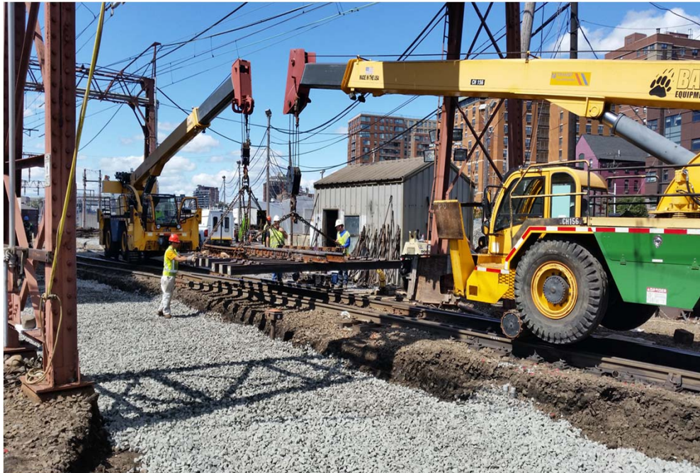
NJ TRANSIT FORCE ACCOUNT EMPLOYEES INSTALLING TURNOUT SWITCH
