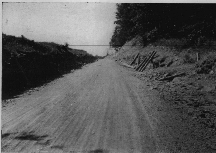
Essex County, Central Avenue and Greenbrook Avenue, Stone Construction, After Improvement. Slopes and shoulders not yet completed.
