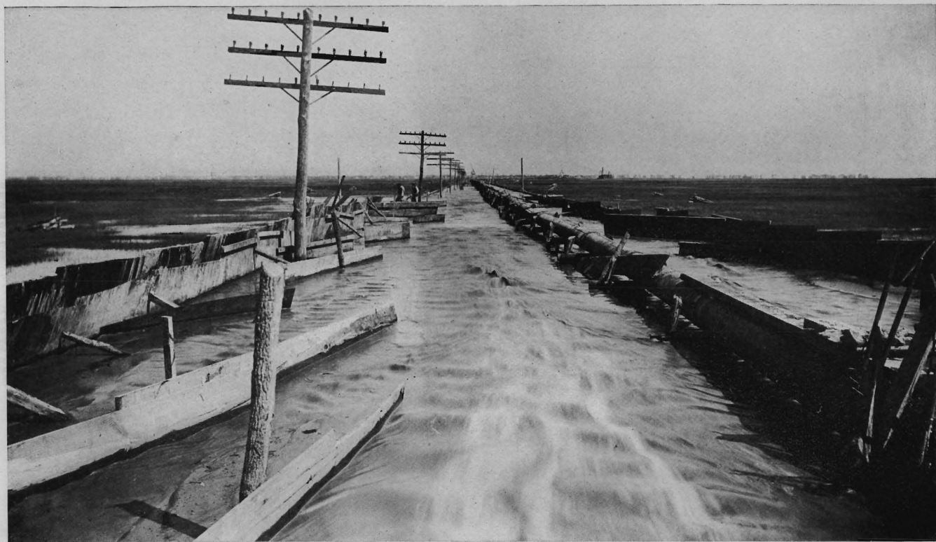
Cape May County, Holly Beach Turnpike, During Construction, Pumping in Sandfill.
