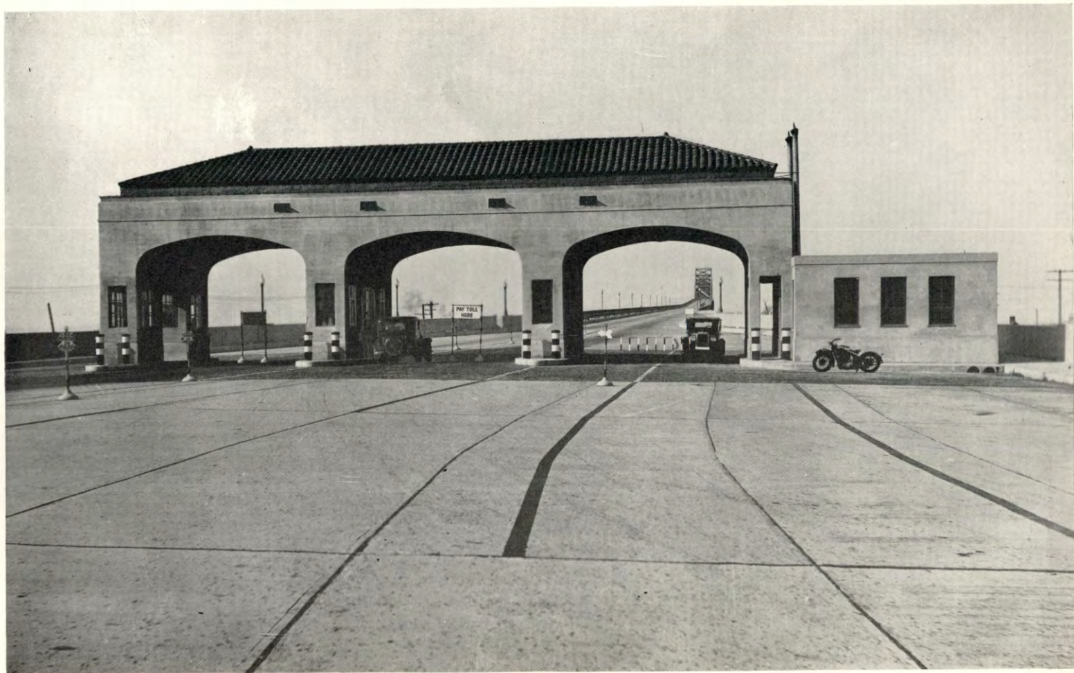
Toll Booth Area, Goethals Bridge
