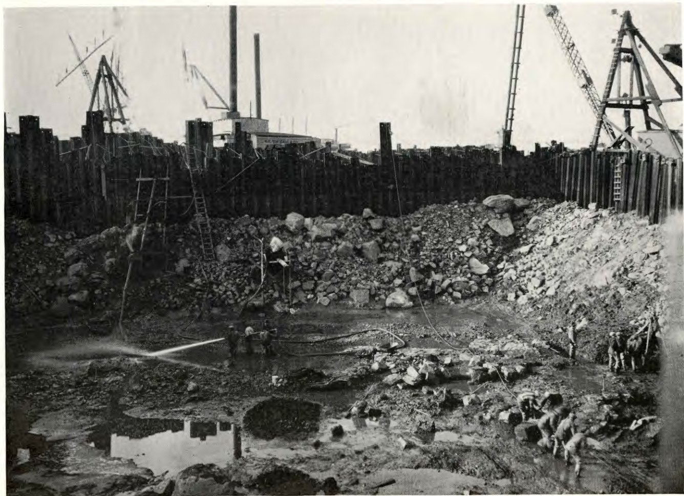
Kill Van Kull Bridge. Inside of Cofferdam—Staten Island Abutment.
