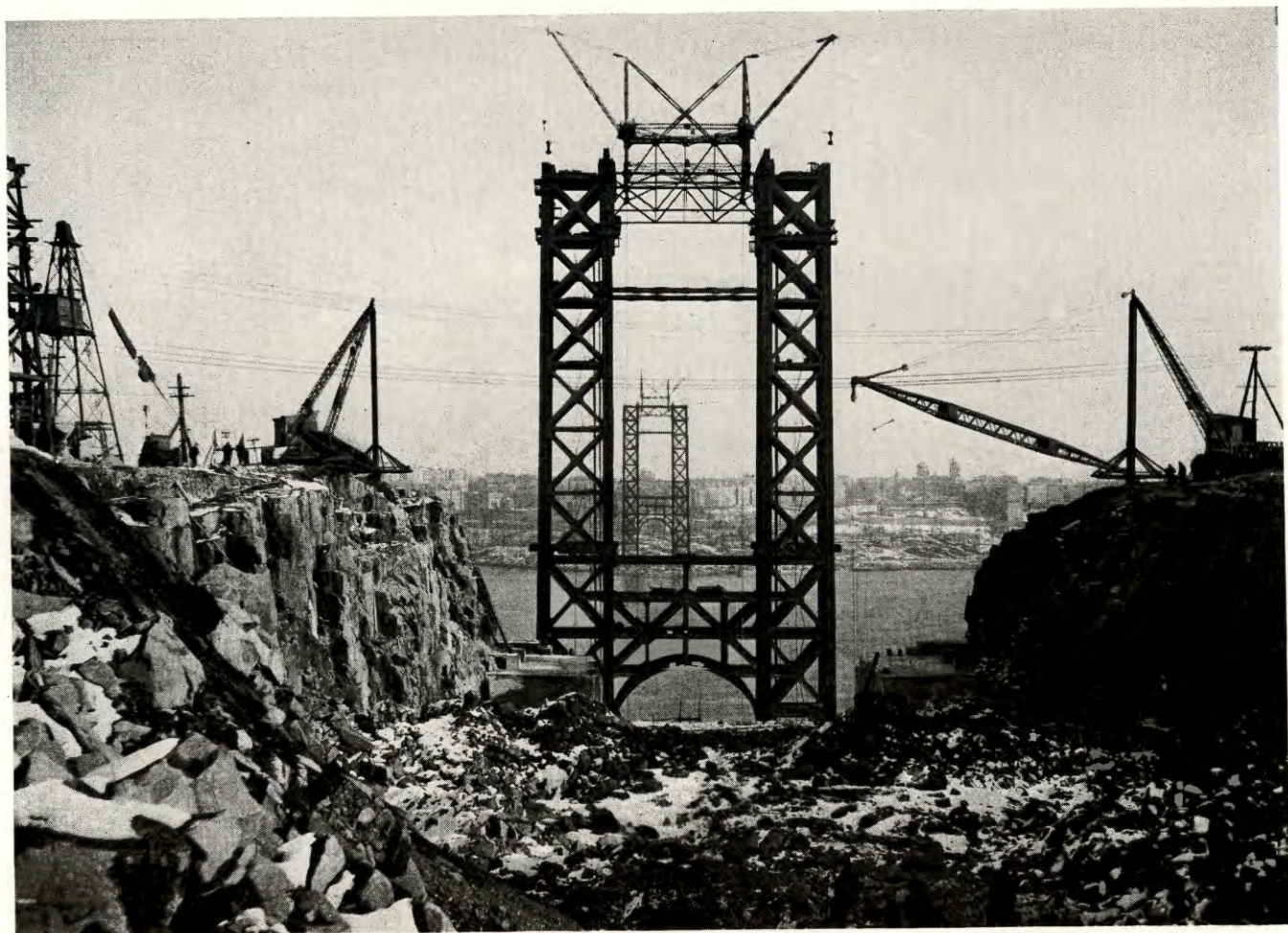
Hudson River Bridge. New Jersey Side. View Looking East Through Rock Cut.
