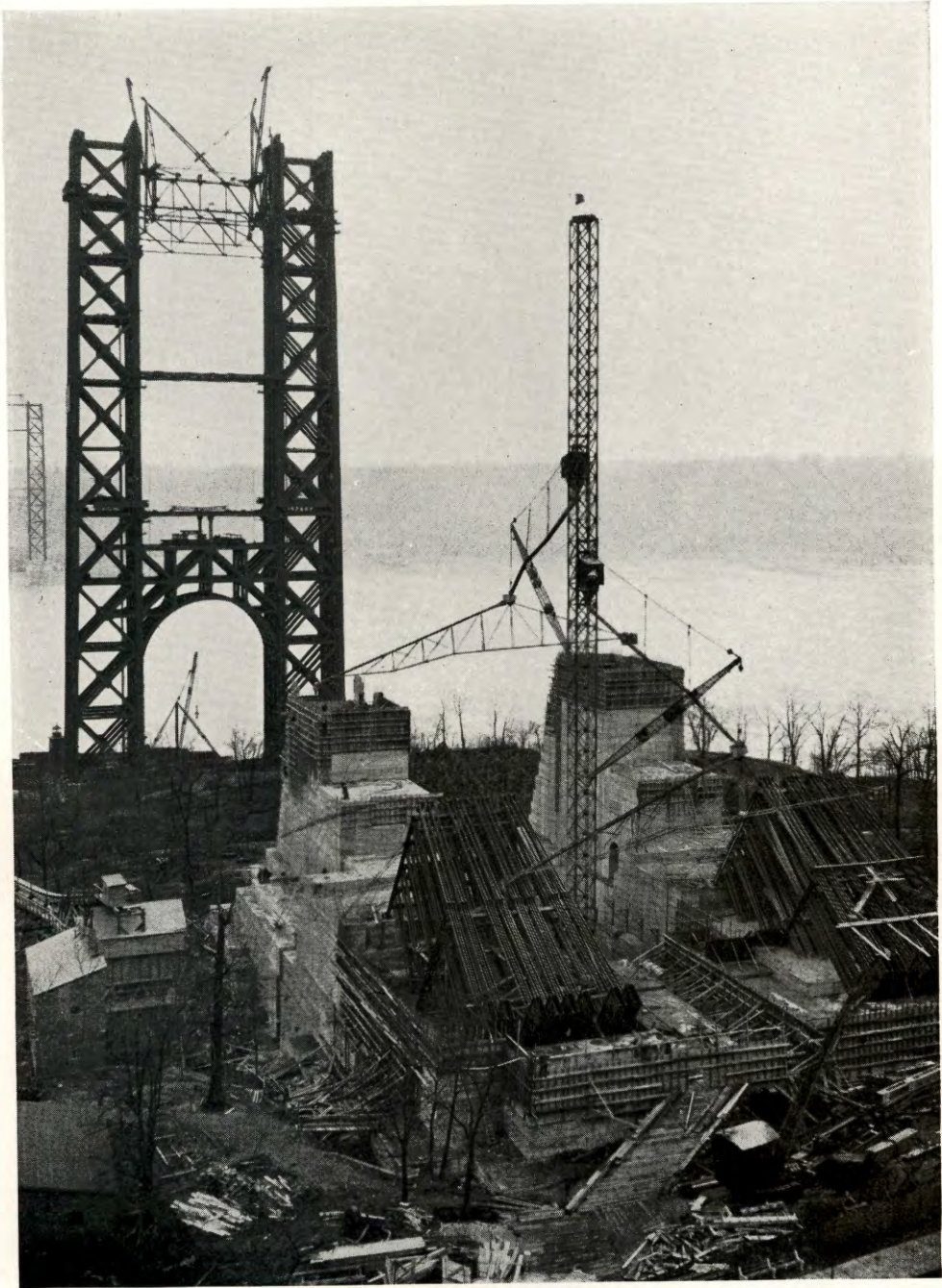
Hudson River Bridge. Construction of New York Anchorage and Tower.
