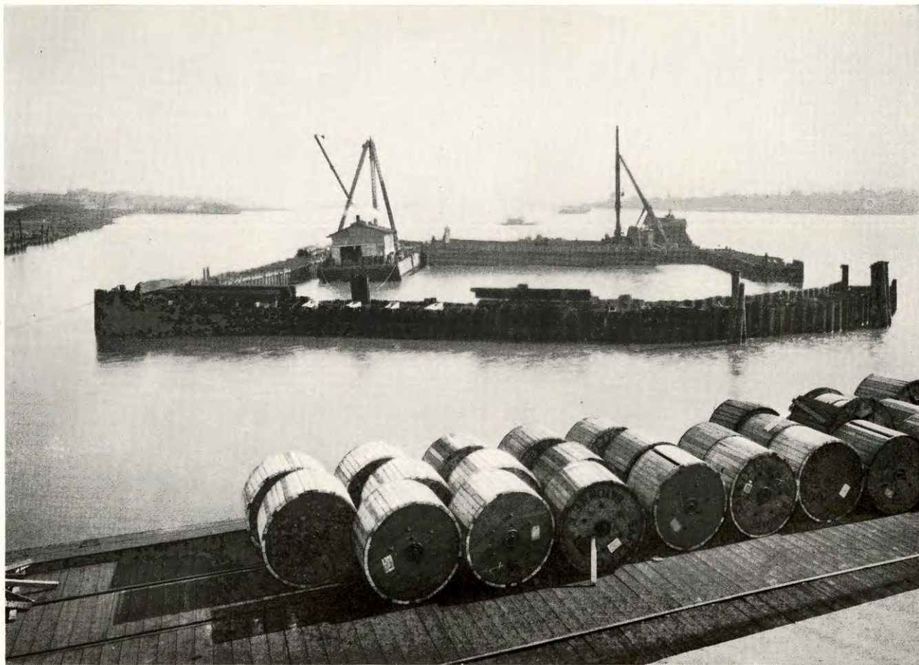
Kill Van Kull Bridge. Construction of Cofferdam—Bayonne Abutment.
