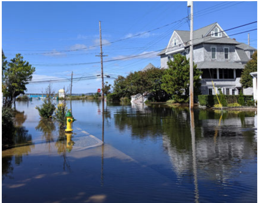
Nuisance Flooding in Seaside Park, NJ
