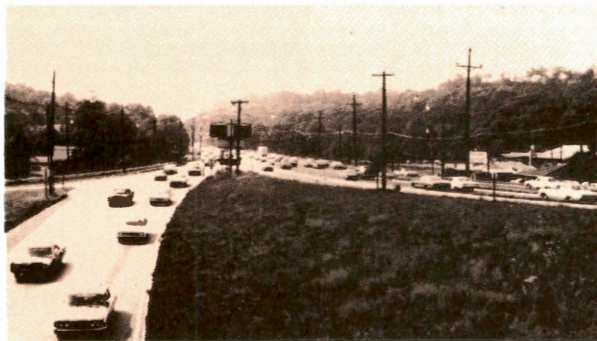
◀ At the juncture of N. J. 3 and U. S. 46, five fully loaded westbound lanes of traffic attempt to merge into three lanes, resulting in a daily bottleneck.
