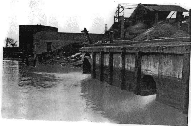
A sewage outfall: discharging raw sewage into the Delaware River.
