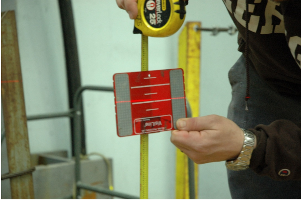
Figure 360. Deck level measurements using laser
