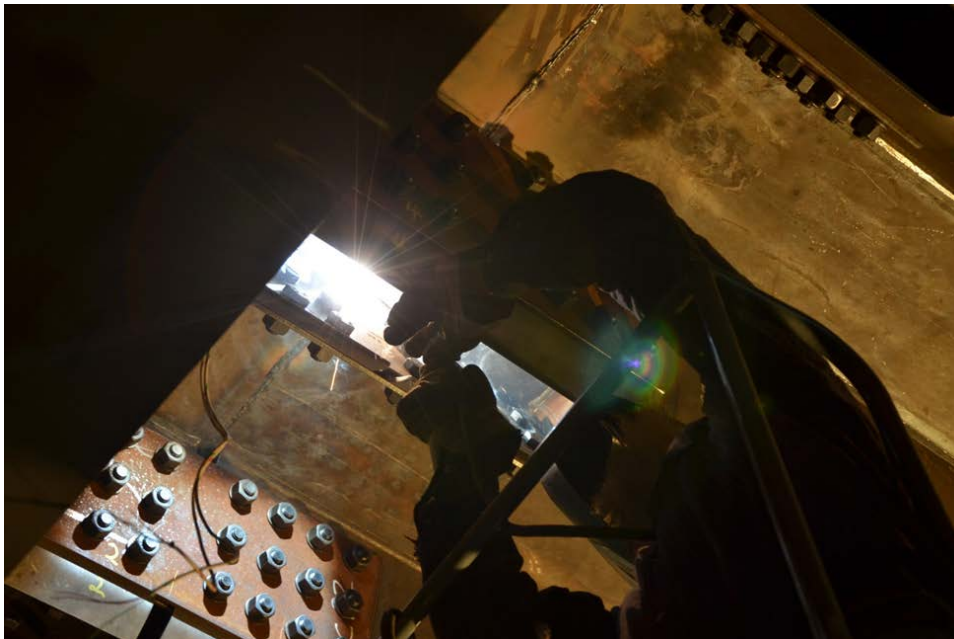
Figure 357. Extensive efforts for back gouge and re-welding inside the rib
