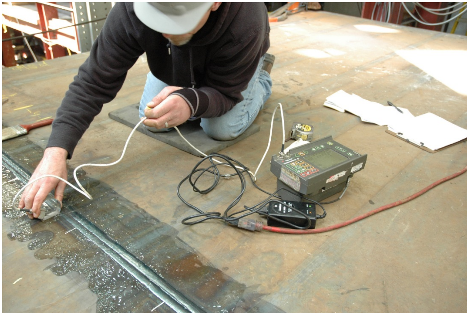
Figure 355. UT of CJP Deck Splice
