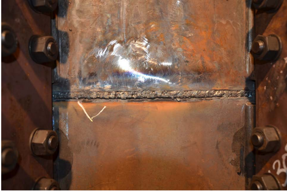
Figure 354. Weld root after removing of backing bar
