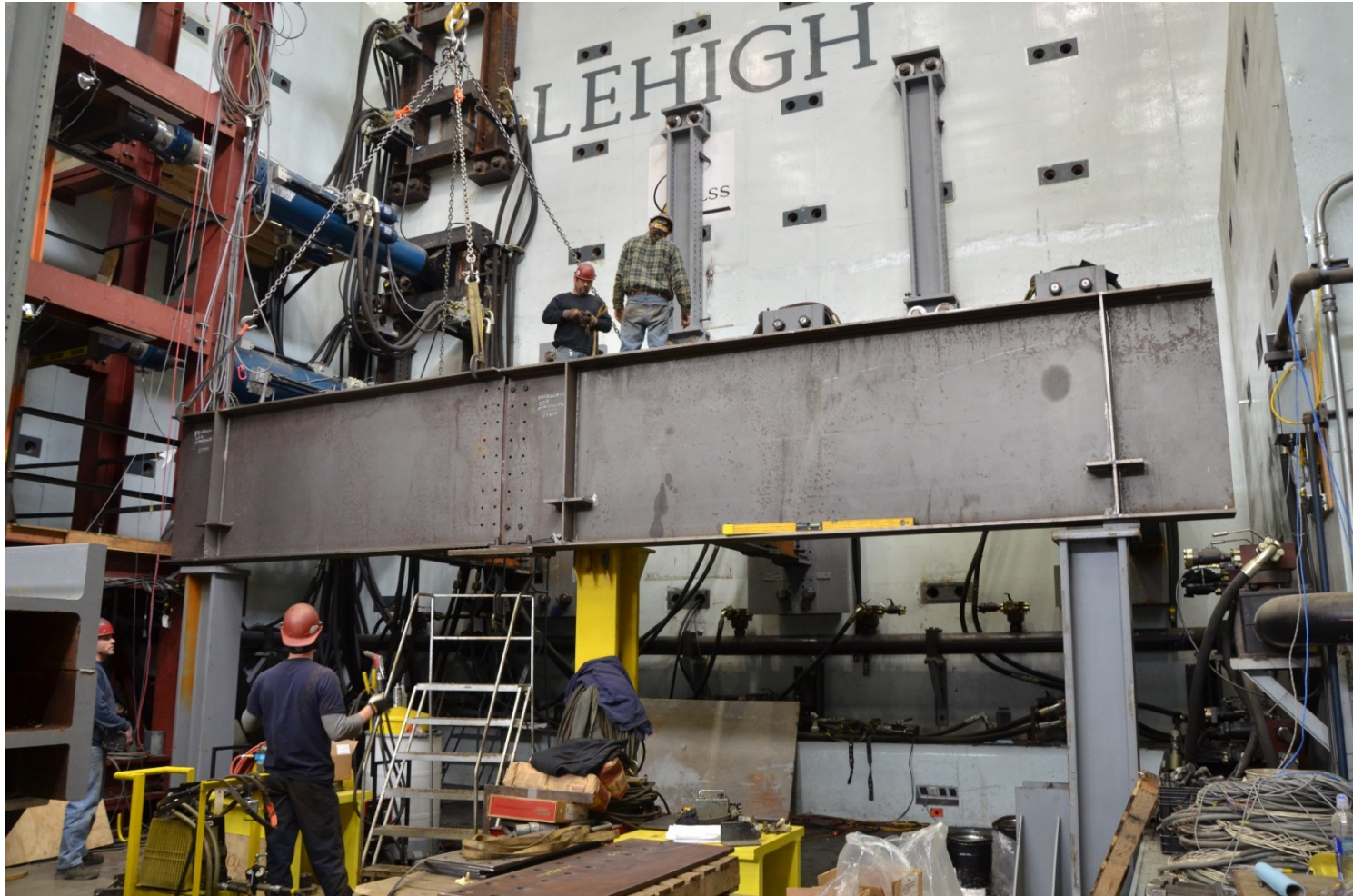
Figure 345. Installation of the west panel
