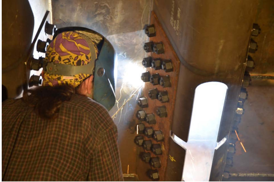
Figure 356. Back gouge and re-welding in between the ribs
