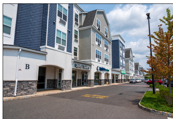
Above: Barnegat 67 in Barnegat Township, Ocean County is a mixed use development project that required the redemption of 9.5 PDCs, or 38 rights. Photo/Paul Leakan
