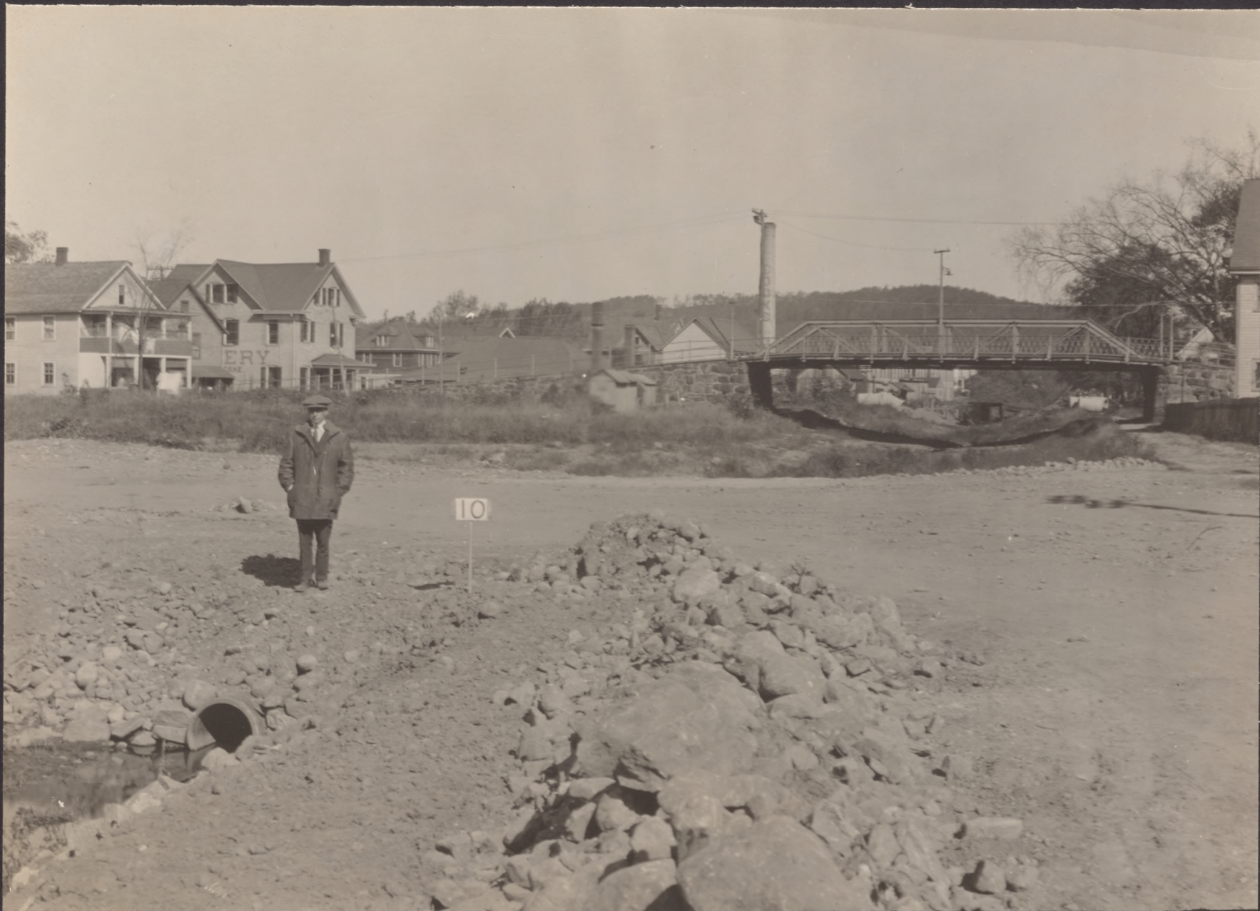
№ 10 FILL IN MORRIS CANAL AT NORTH BERGEN ST DOVER VIEW LOOKING SOUTH EAST OCT 10, 1924
