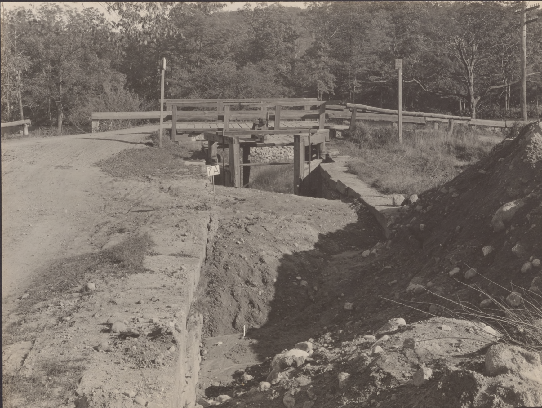
Nº 7A FILL IN LOCK OF MORRIS CANAL WEST OF ROCKAWAY RIVER AT POWERVILLE ABOVE BOONTON VIEW LOOKING EAST TOWARD BRIDGE #84 - OCT. 9, 1924
