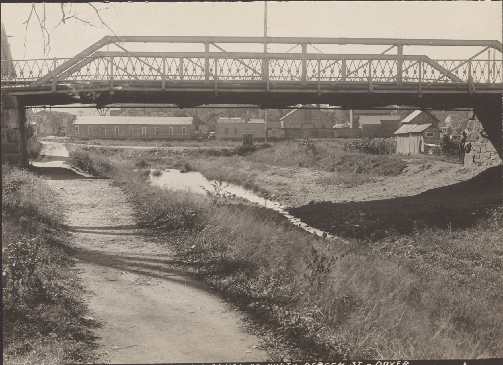
Nº 10 B FILL IN MORRIS CANAL AT NORTH BERGEN ST. - DOVER VIEW LOOKING NORTH WEST OCT. 10, 1924
