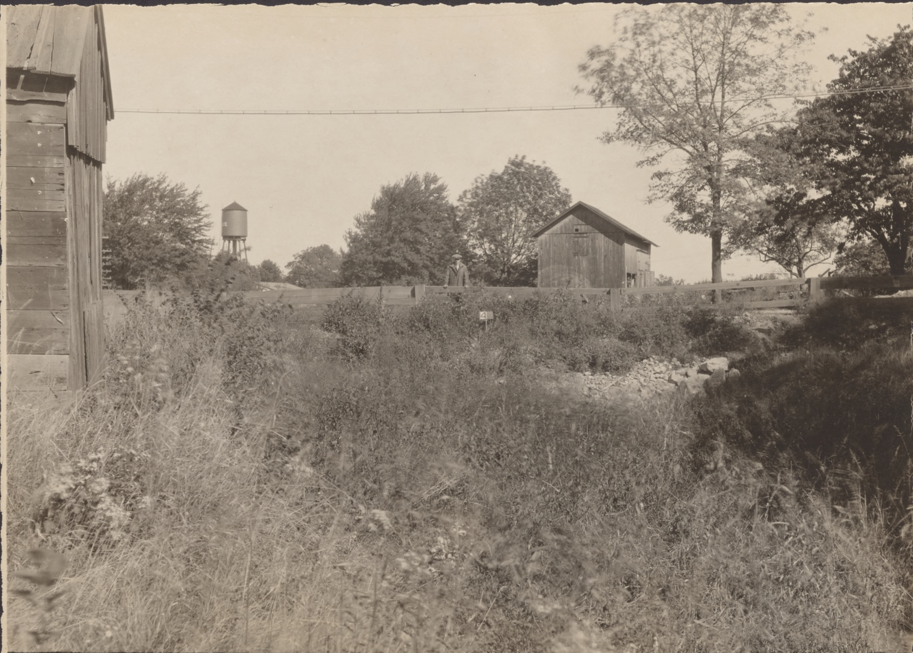
N o 4. FILL IN MORRIS CANAL AT SITE OF VREELAND AVENUE BRIDGE - BOONTON VIEW LOOKING SOUTHEAST OCT 9, 1924
