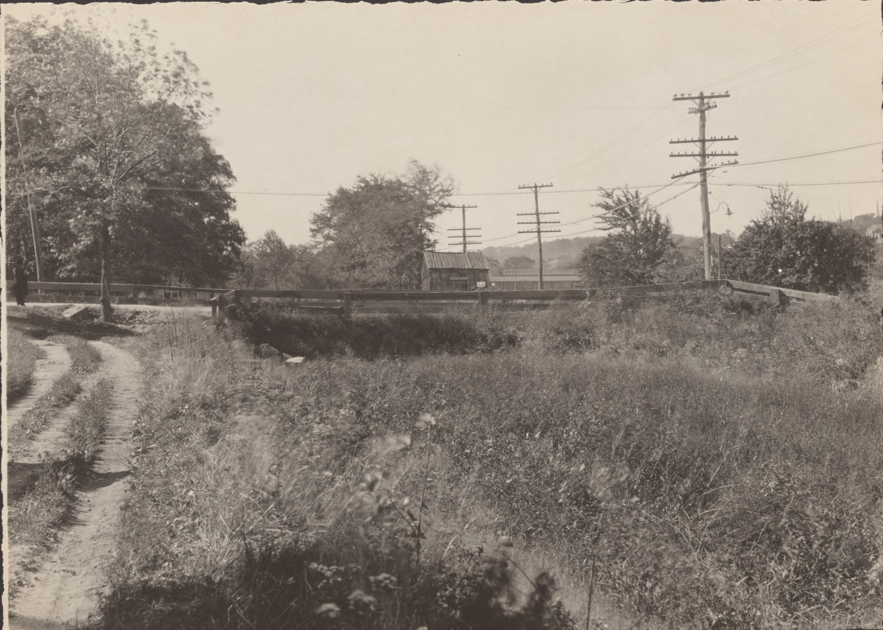
NO 4A FILL IN MORRIS CANAL AT SITE OF VRELAND AVENUE BRIDGE - BOONTON VIEW LOOKING NORTH WEST OCT 10, 1924
