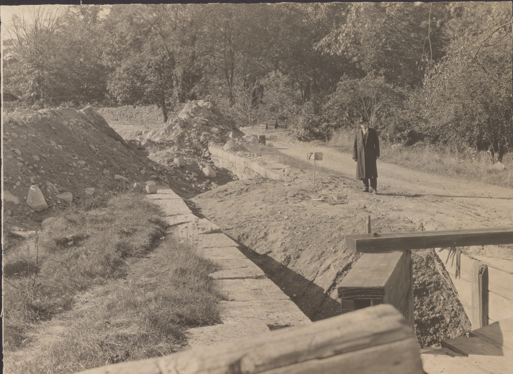
N o 7 FILL IN LOCK OF MORRIS CANAL WEST OF ROCKAWAY RIVER AT POWERVILLE ABOVE BOONTON VIEW LOOKING WEST FROM BRIDGE #84 - OCT. 9, 1924
