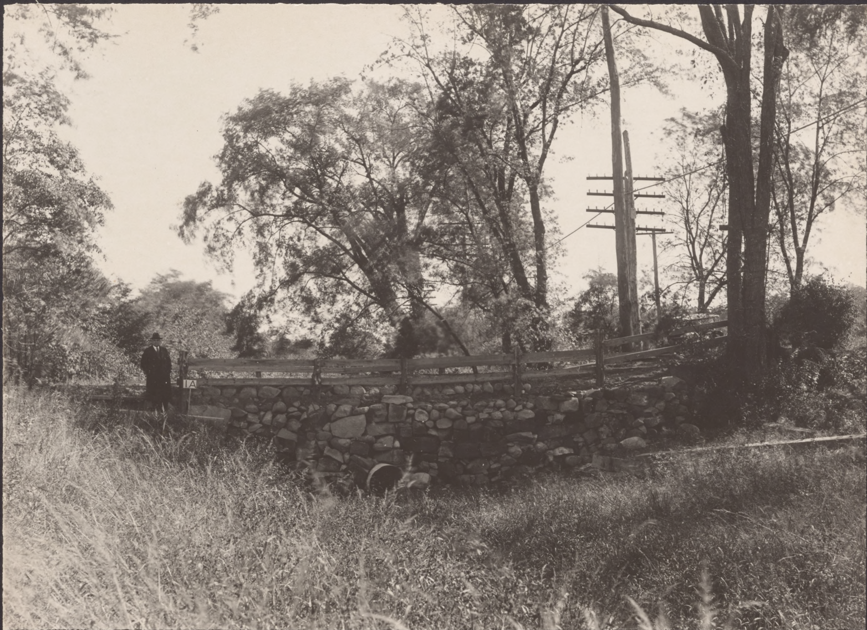
N o 1A SITE OF RYERSON BRIDGE ON MORRIS CANAL 8 1/10 MILES NORTH OF ACQUEDUCT AT MOUNTAIN VIEW VIEW LOOKING SOUTH
