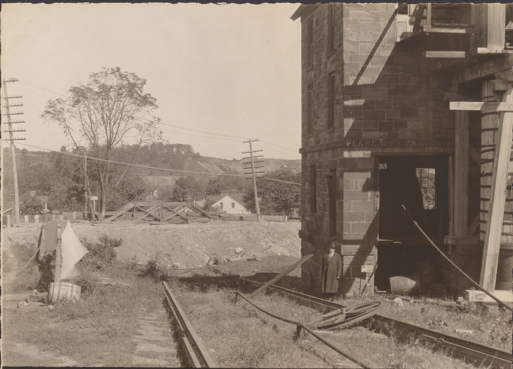
No 3 FILL AT MAIN ROAD CROSSING OF MORRIS CANAL ON PLANE #9 EAST AT MONTVILLE VIEW LOOKING SOUTH EAST OCT. 9, 1924
