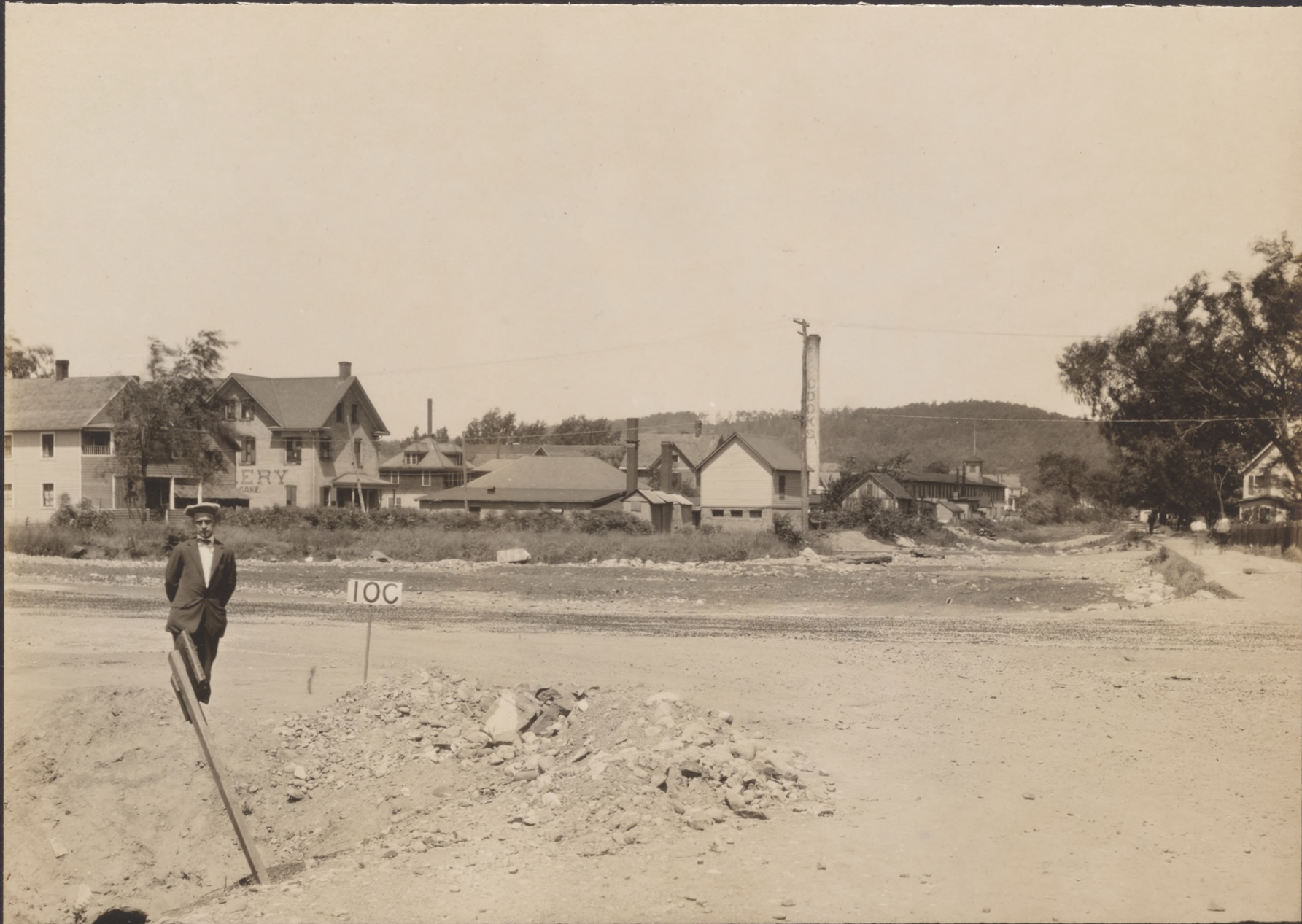
NO 10 C SAME LOCATION AS NO. 10 SHOWING SITE OF HUDSON ST BRIDGE AND FILL IN CANAL BED BETWEEN HUDSON ST AND NORTH BERGEN ST AT DOVER JUNE 11, 1925
