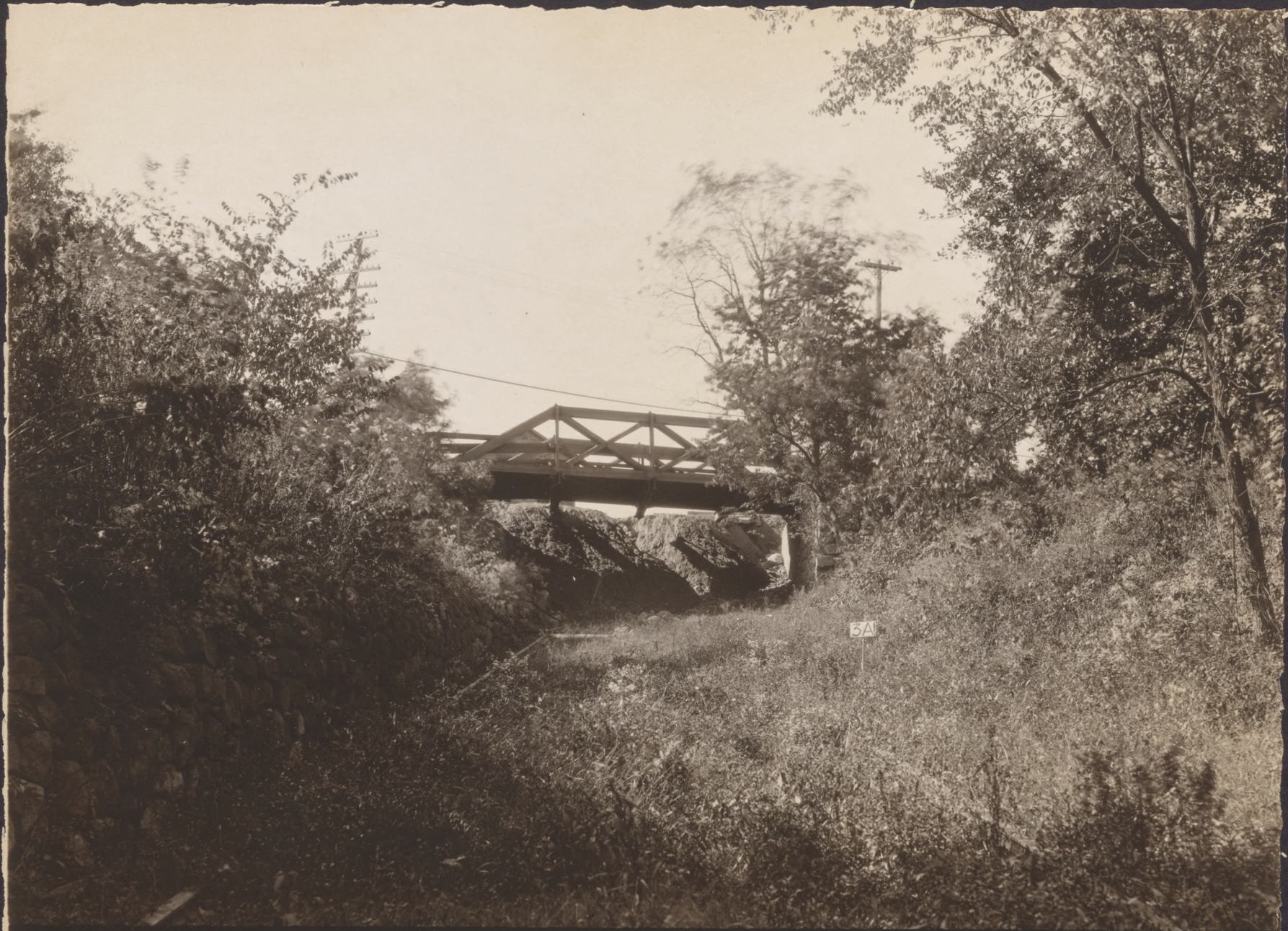
NO 3A FILL AT MAIN ROAD CROSSING OF MORRIS CANAL ON PLANE #9 EAST AT MONTVILLE VIEW LOOKING NORTH WEST OCT. 10, 1924
