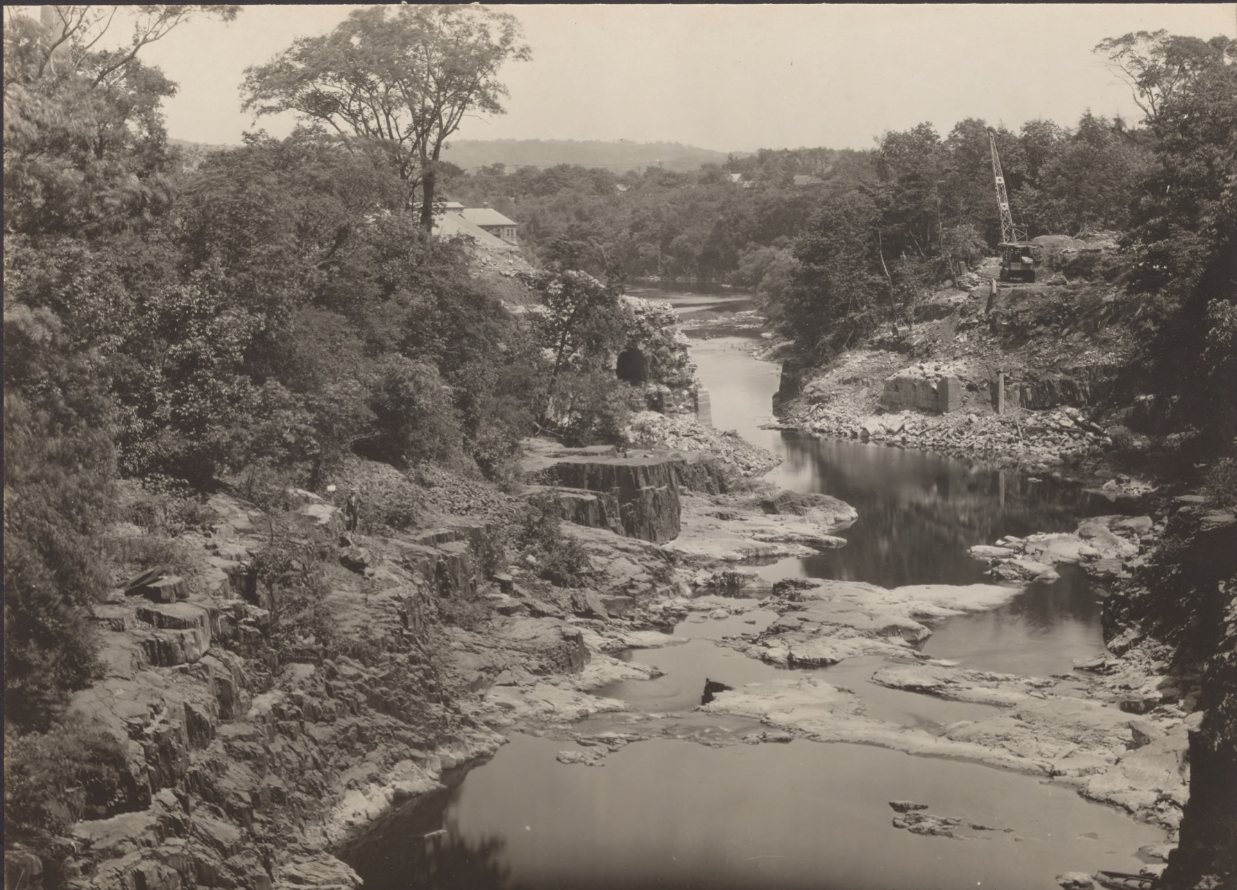
NO. 12 SITE OF MORRIS CANAL AQUEDUCT, CROSSING PASSAIC RIVER AT LITTLE FALLS VIEW LOOKING DOWNSTREAM
