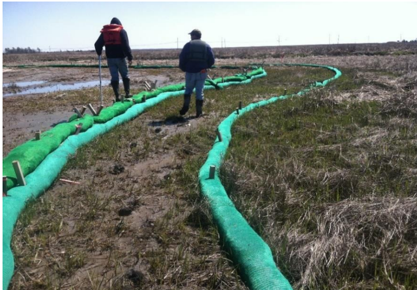
Figure 34. At Fortescue, the team installed Filtrexx SiltSoxx™ containment in two concentric rows along the perimeter of the dredged material placement areas.
