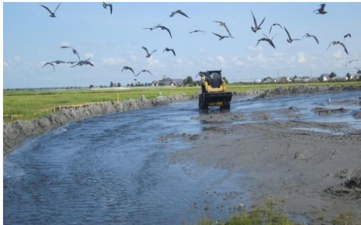
Figure 24. A front-end loader was used to move the sand during pumping and after dewatering.
