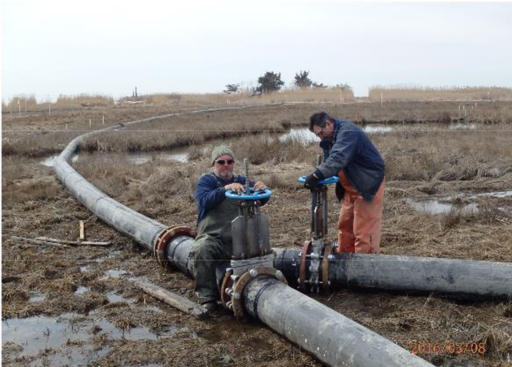
Figure 37. This y-valve allowed the team to change the location of sediment placement without moving the pipe. Photo from Dewberry Engineers Inc., courtesy of NJDOT.
