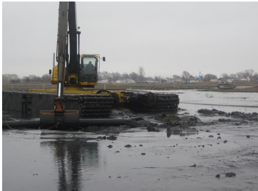
Figure 39. At Fortescue, an excavator held and repositioned the dredge discharge pipe outlet.
