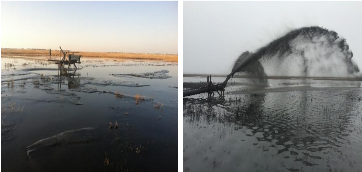
Figure 32. The dredge pipe outlet at Avalon, Phase 2, was fitted with either a spreader plate (left) or a spray nozzle (right).
