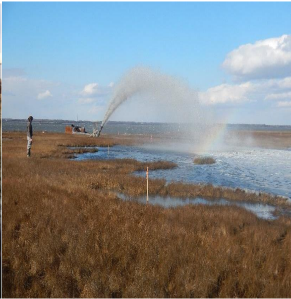
Figure 26. At Avalon, grade stakes helped indicate elevations about the marsh surface during dredged material spraying.
