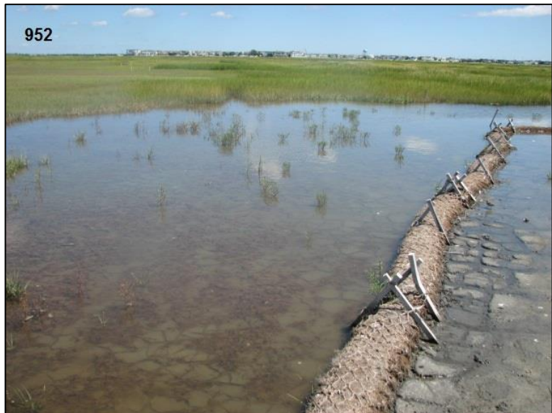
Figure 51. At Avalon Phase 2, vegetation die-off (brown areas outside containment) occurred (top). The containment restricted tidal flow, keeping water higher outside the placement area than inside it. Photos from NJDEP.
