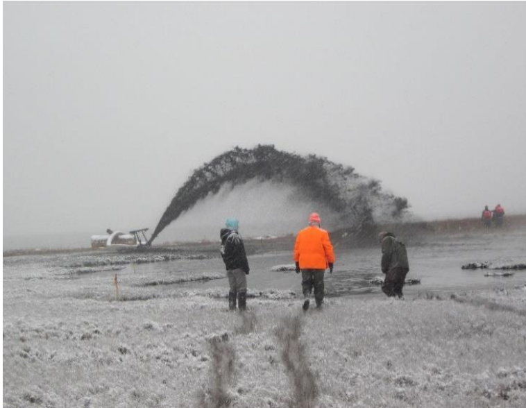
Figure 27. At Avalon, dredged material spraying in placement area A used the lessons learned from work at placement area C.
