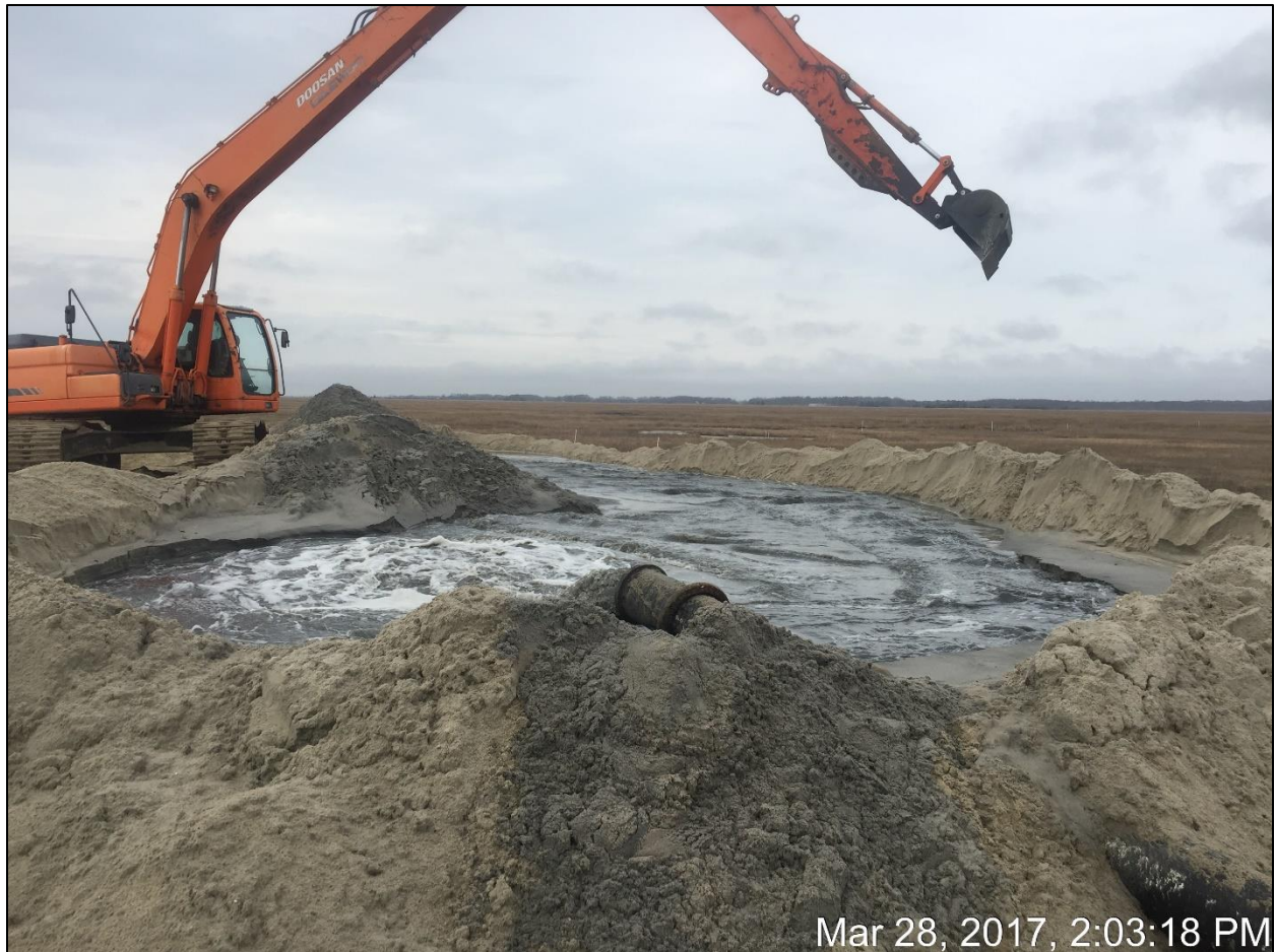
Figure 41. At the Fortescue dune restoration, berms were constructed from the first dredged sediment to create dewatering pits to retain the dredged material and to direct the dewatering discharge to the center of the placement area. Photo from NJDOT.
