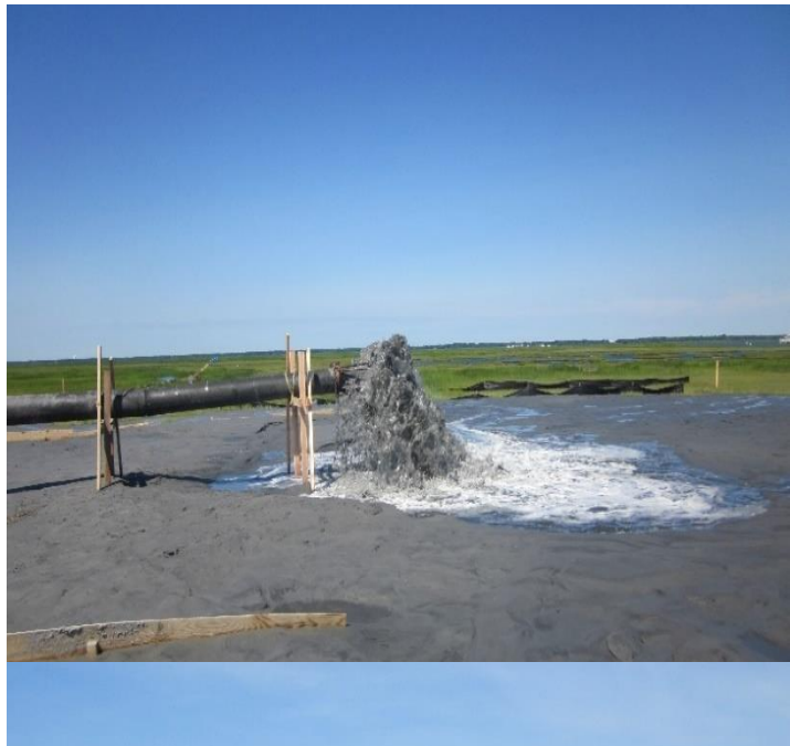
Figure 23. Containment measures were placed around the Ring Island Enhanced Nesting Habitat site.
