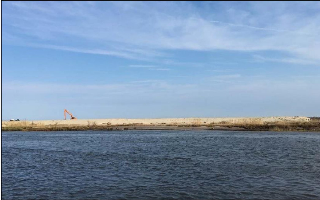
Figure 41. This photo of the Fortescue dune restoration shows the bay side of the dune immediately after placement.
