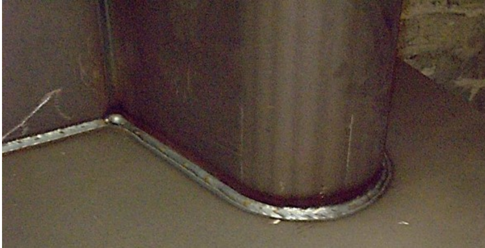
Figure 323. Rib-to-deck plate welding
