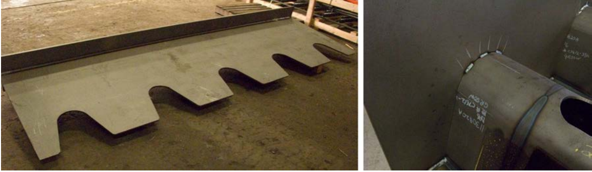
Figure 331. Match-cutting of floor beam for rib-to-floor beam weld
