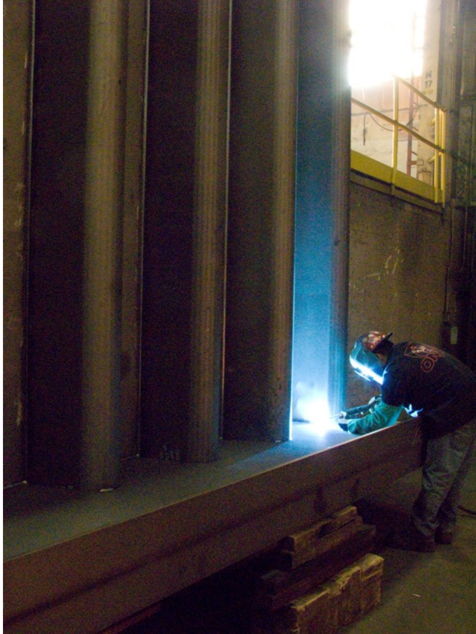
Figure 333. Rib-to-floor beam welding in 2F position
