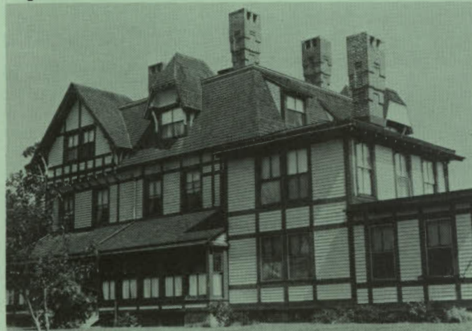
Historic Site Restoration, Physick Estate, Cape May
