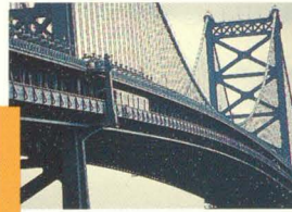
BENJAMIN FRANKLIN BRIDGE
