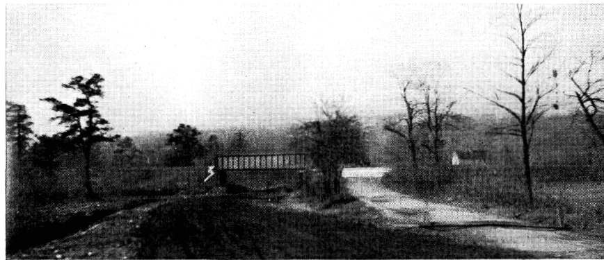
FIG. 21—Highway diverted to canal bed, and a railroad grade crossing abolished.
