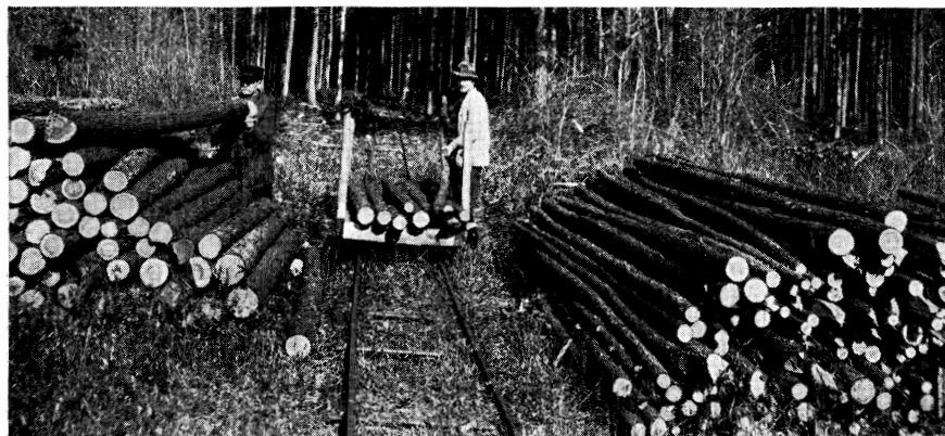
FIG. 10—Portable track for swamp logging and cedar thinning on Lebanon Forest.
