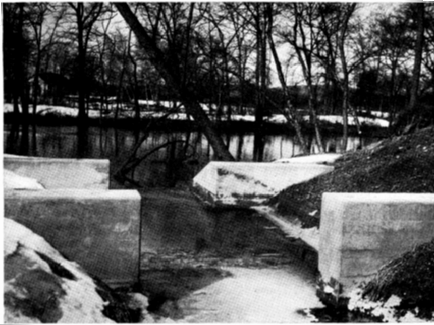
FIG. 22—Drainage cut, Pompton Feeder into Pompton River.
