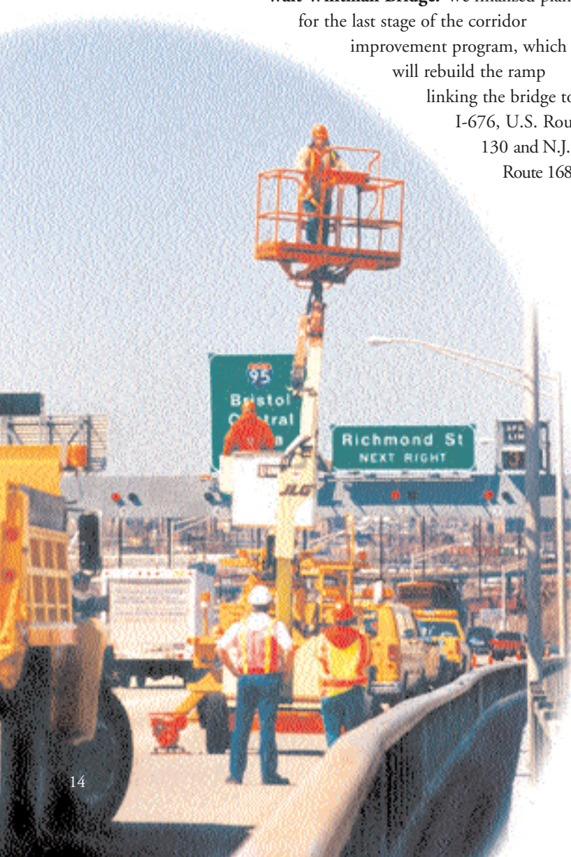
◀ Maintenance crews at the Betsy Ross Bridge.
