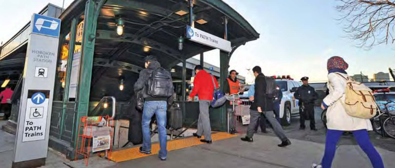
During Superstorm Sandy, saltwater flooded the Hoboken tunnels, compromising the electrical system and other equipment. Repairing the system required complicated staging operations.
