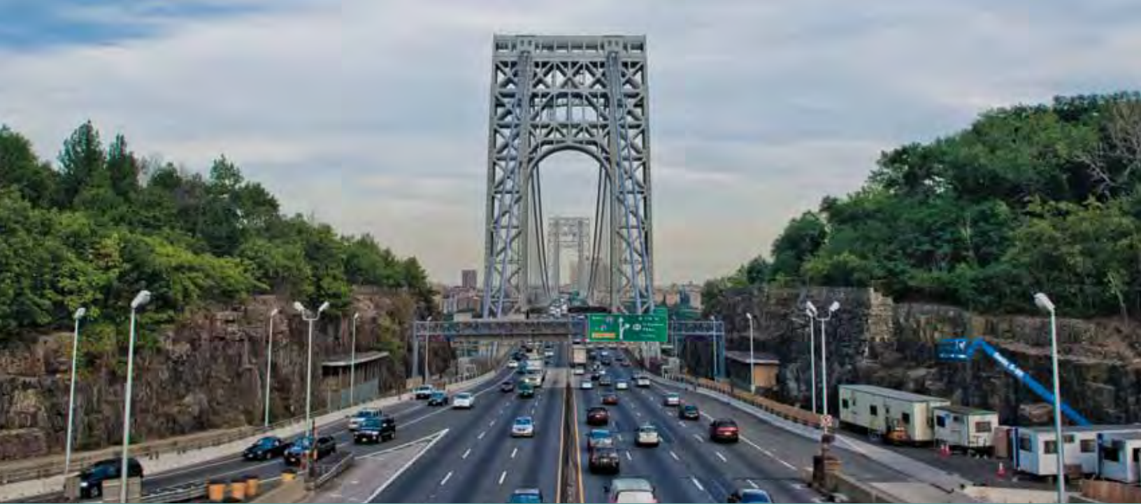
The George Washington Bridge carries approximately 102 million vehicles per year, making it the world's busiest motor vehicle bridge.
