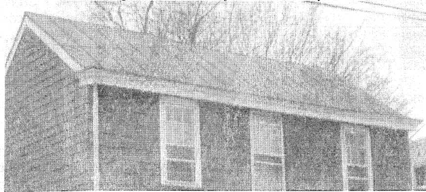
Standing seam metal roof at 204 Barclay Street
