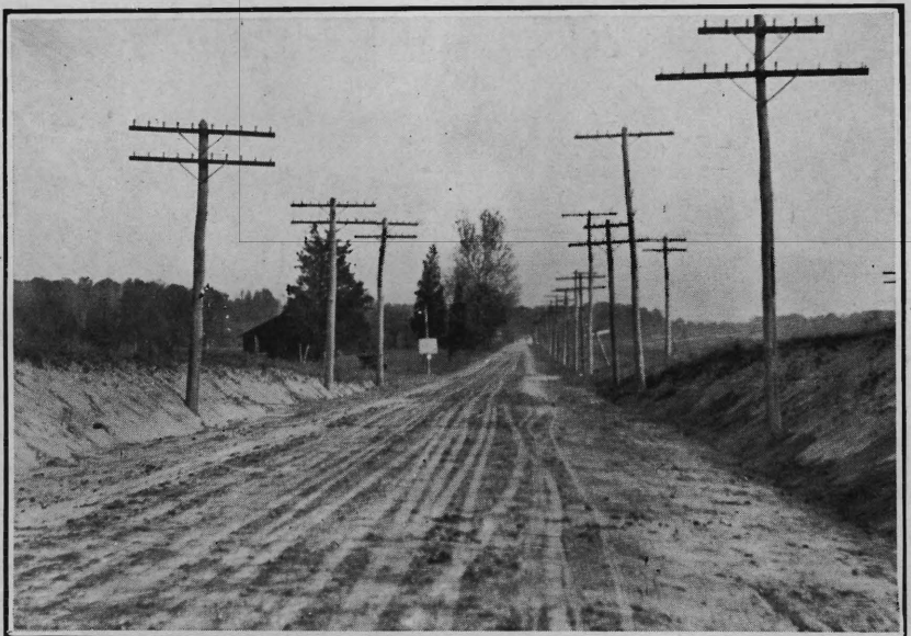
Yardville-Newtown-Windsor Road, Mercer County, After Improvement.
