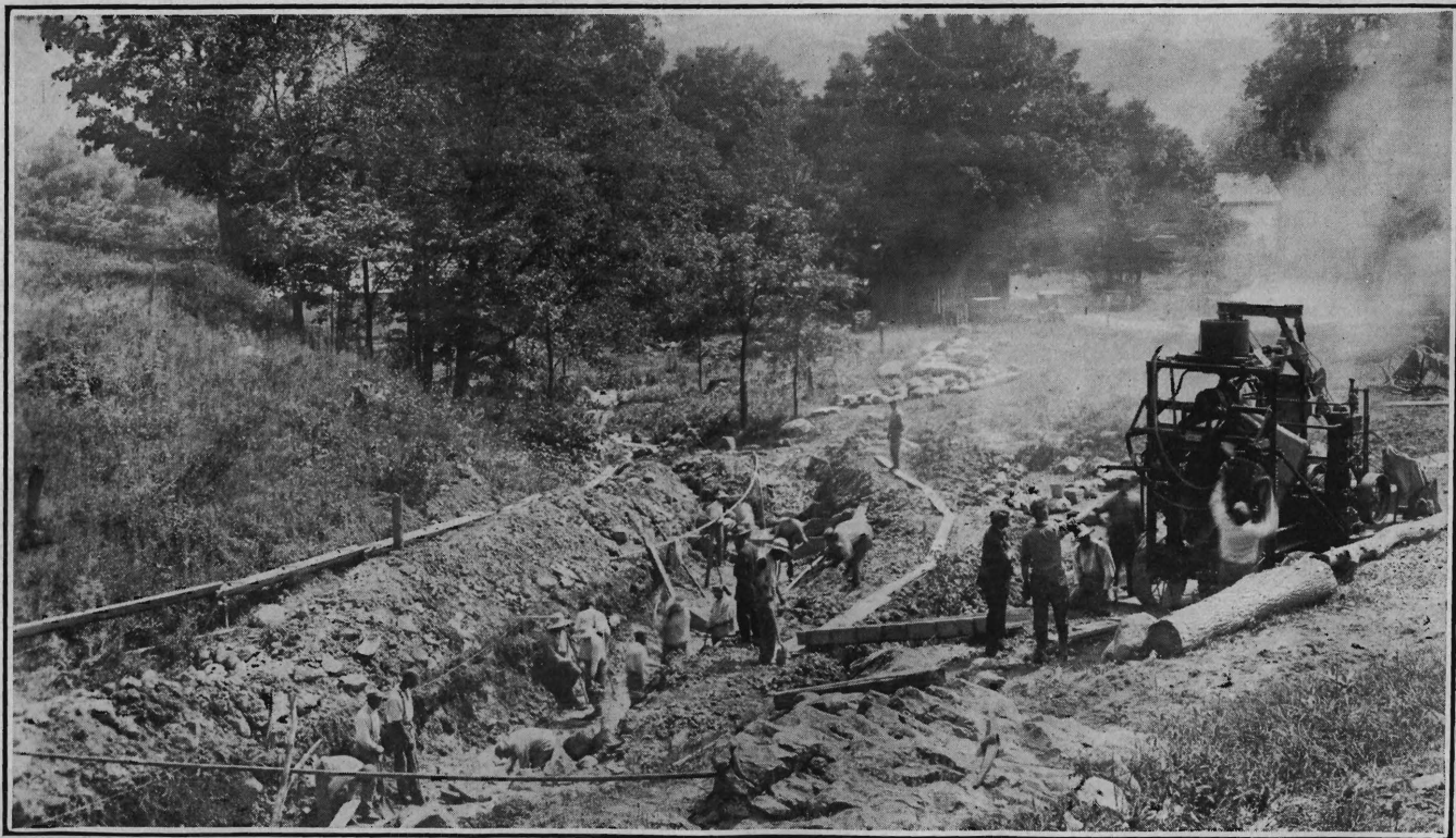
Convict Labor, Camp No. 1B, Layton-Dingman's Road, Construction Work.
