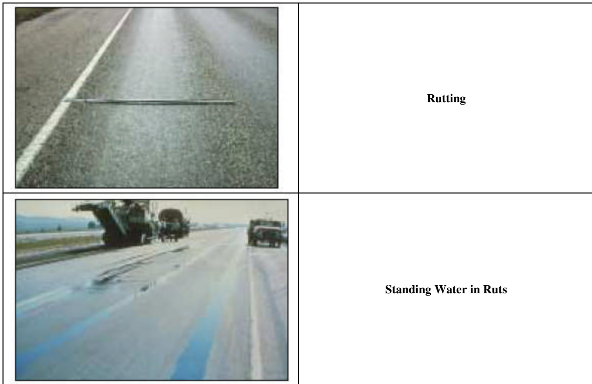
Figure 14. Illustration of Pavement Wheel Track Rutting
