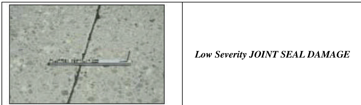
Figure 20. JOINT SEAL DAMAGE
