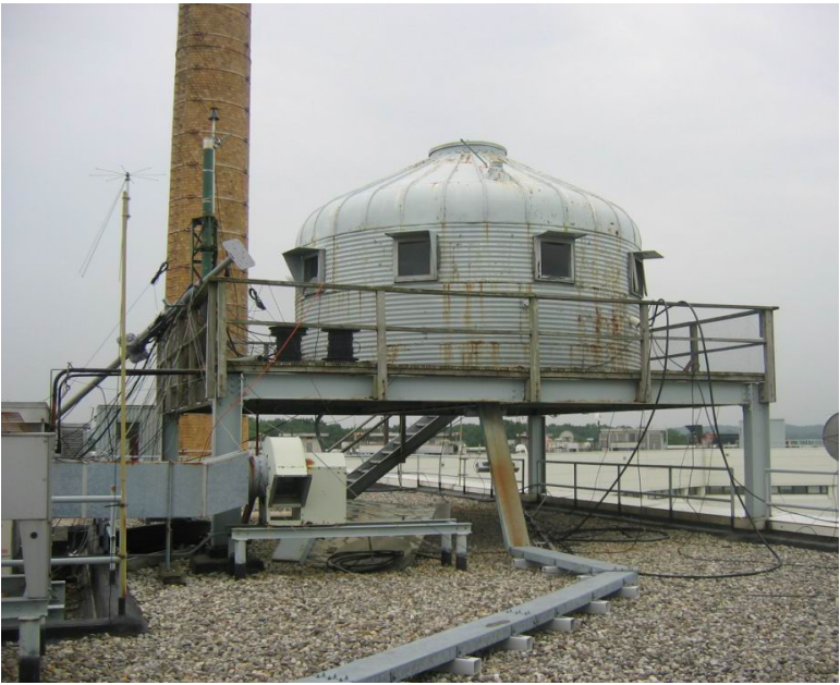
The Dymaxion Deployment Unit should be placed on a concrete foundation, and all materials restored to their original condition.
