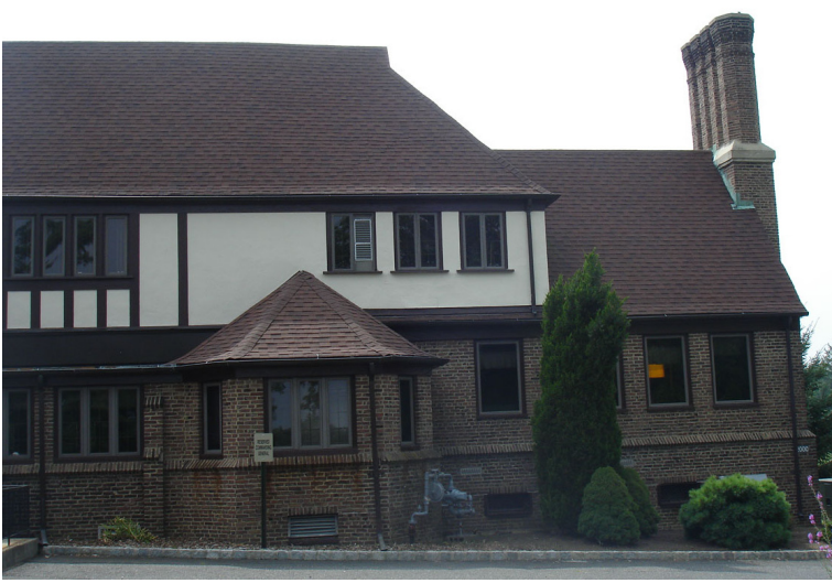
Gibbs Hall, Building 2000
