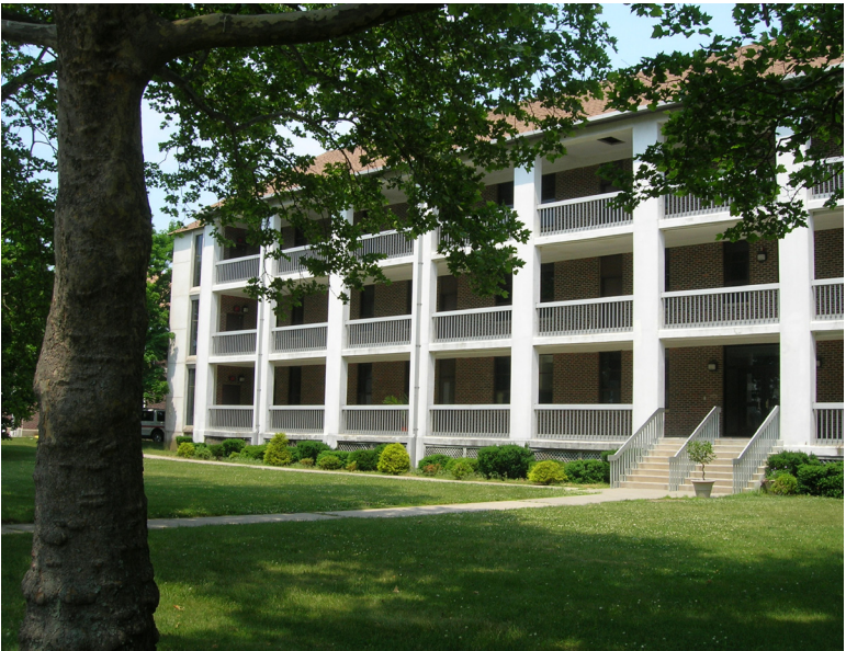
Colonnaded Facade at Barker Circle
