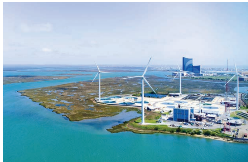
Aerial View of the Jersey-Atlantic Wind Farm. The Trump administration is preventing similar clean energy projects from developing. Photo credit by Drones Flown
