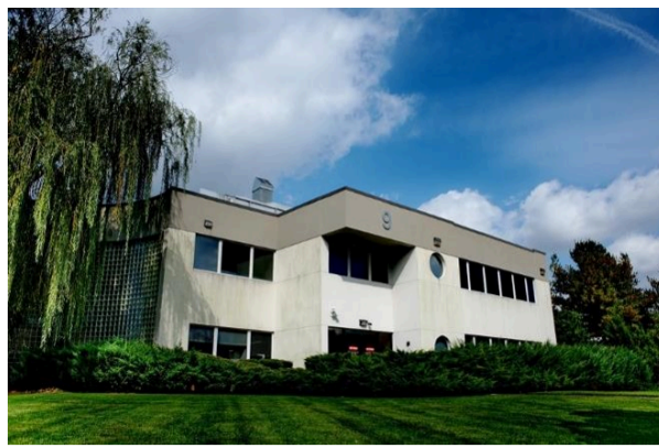
BioCentriq Pilot Plant Deer Park, Building 9
